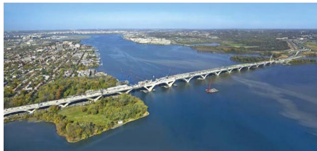
Figure 5.3.8: Concrete V-Piers (Woodrow Wilson Bridge)
