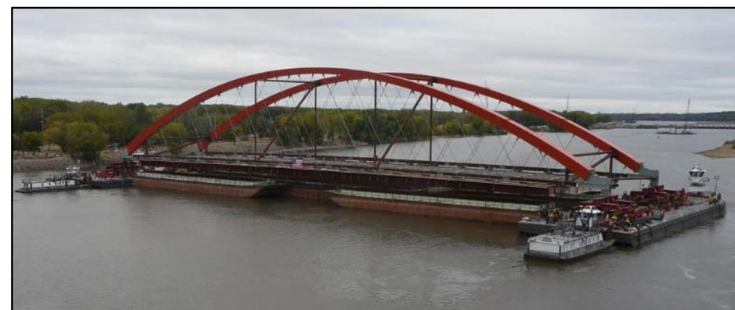
Figure 8.16.6.1: Erection of Hastings Bridge Using SPMT
