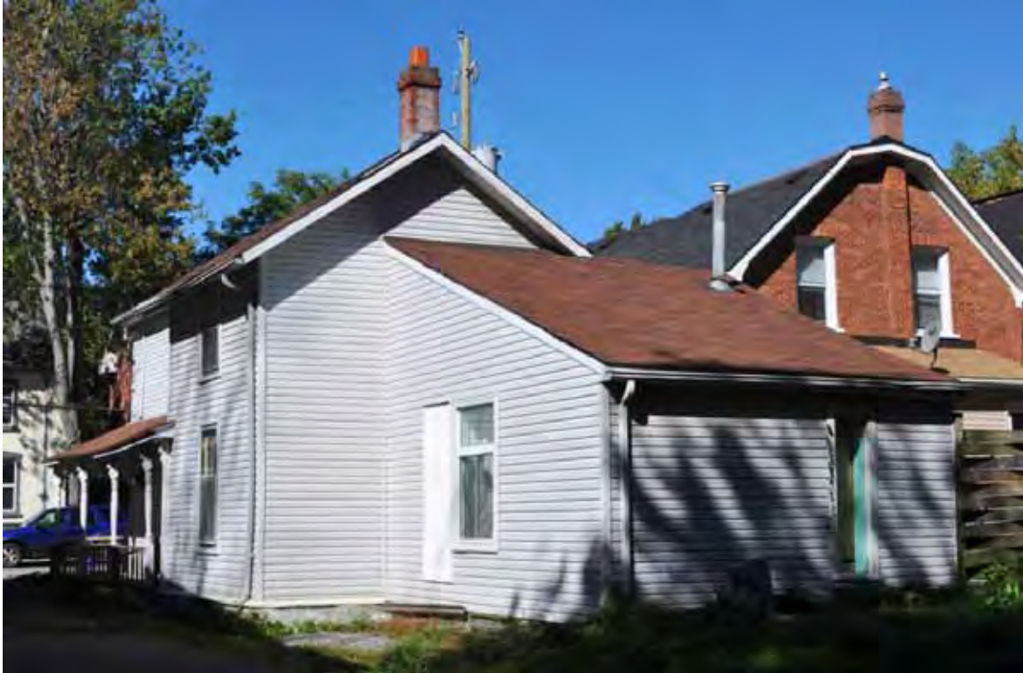
East view of rear façade
