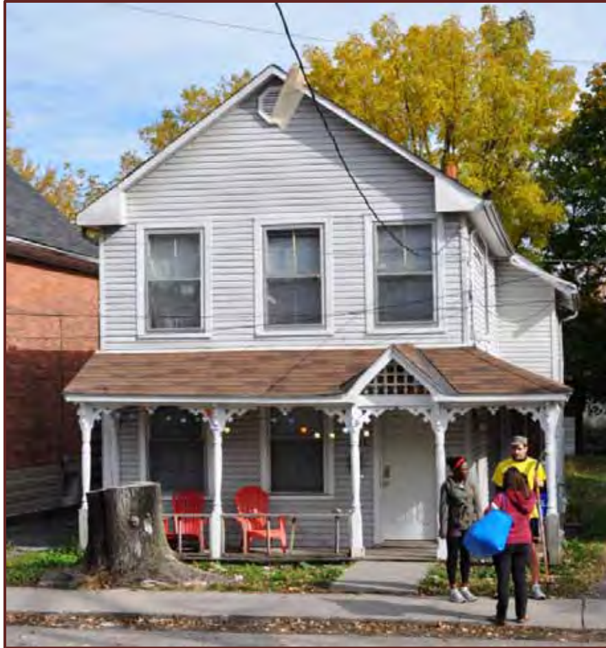
Principal facade facing west; all visible surfaces are covered with modern materials; frame construction
