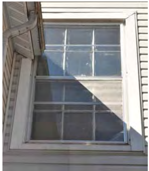
East corner of the main house showing the only surviving original window glazing bars (6 over 6)
