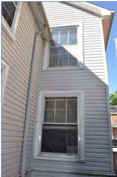
East corner of the main house showing the only surviving original window glazing bars (6 over 6)
