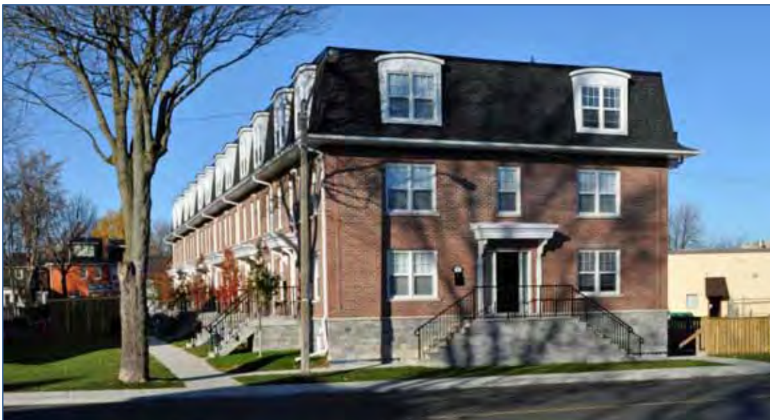
326 Alfred Street, an example of a mansard roof forming the top storey in a modern building
