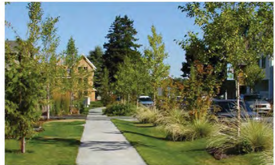
Green street with swale for stormwater and generous landscaping (Seattle).
