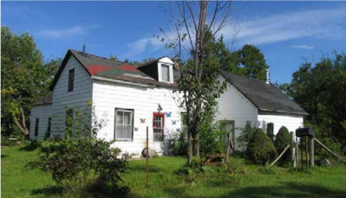
Facing west. Photo by J. McKendry
