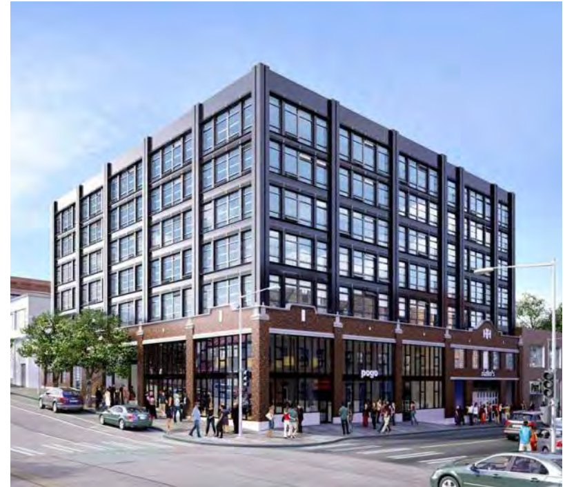
Figure 3-13: Corner building addressing both streets
