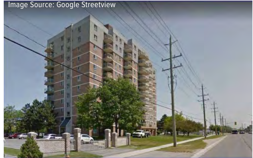
Figure 2-6: Typical apartment building on Bath Road in Hillendale
