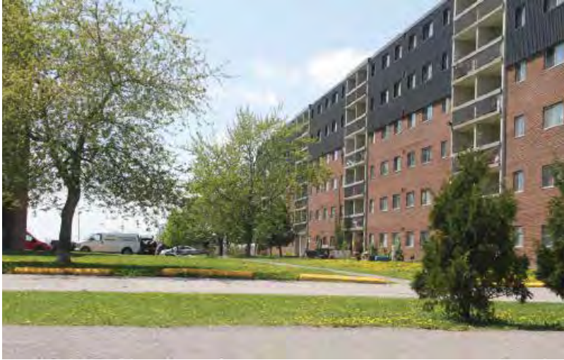
Figure 2-23: Six storey apartment buildings with parking at side in Group 6
