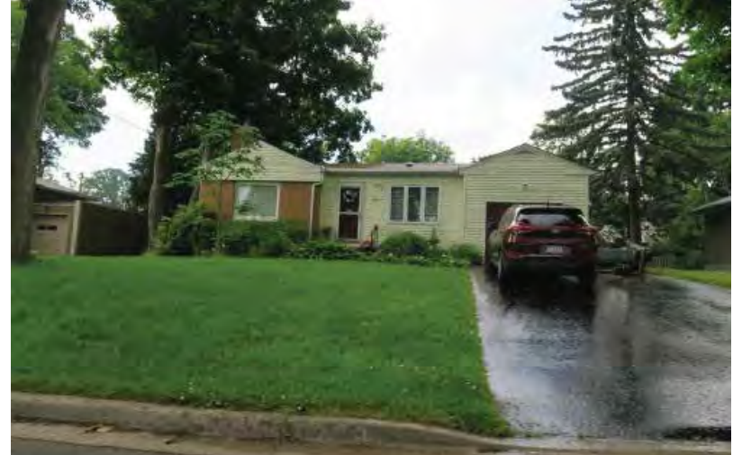
Figure 2-9: Typical single detached house in Group 2
