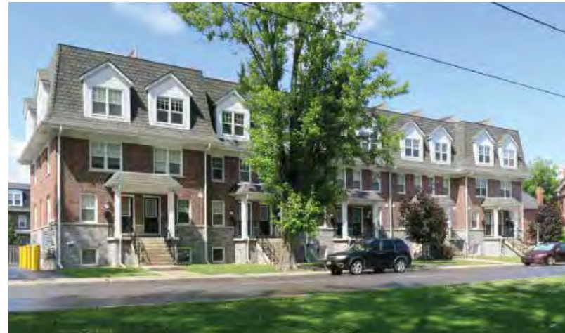
Figure 2-17: Newer development project with a rhythm of front doors, porches and roof dormers in Group 4
