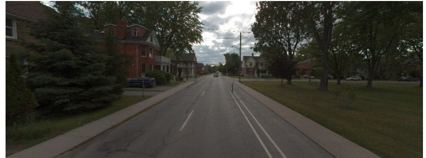
Figure 11. Example of Very Poor Road (OCI 20-0)
