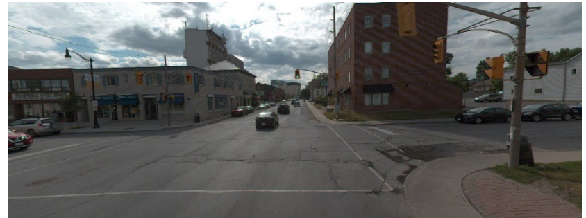
Figure 11. Example of Very Poor Road (OCI 20-0)
