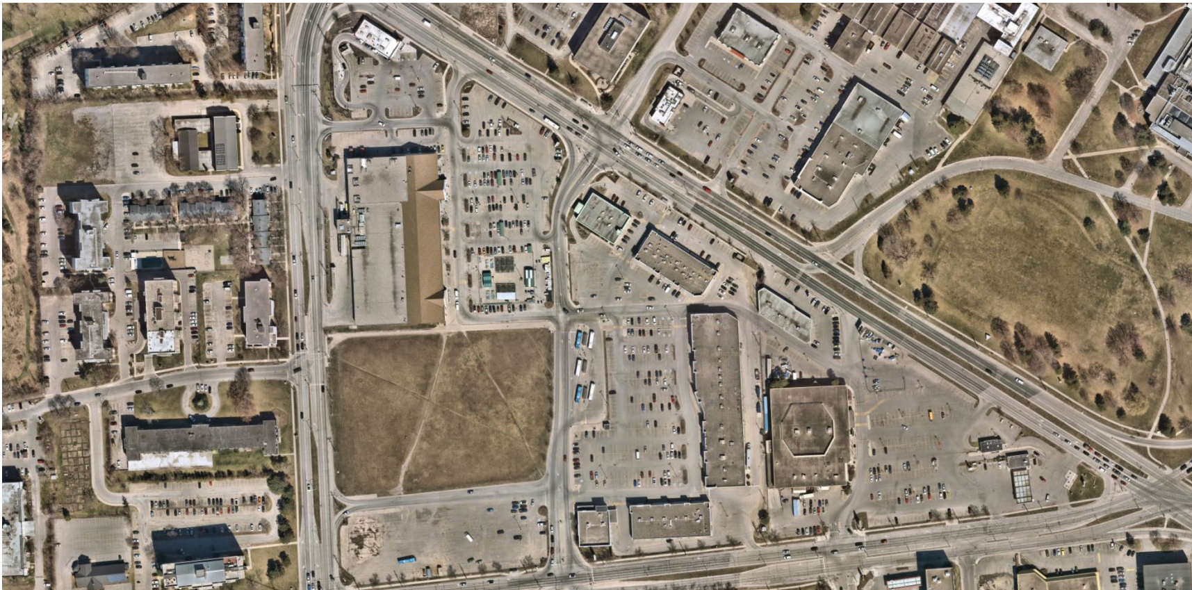
Aerial Image of Kingston Centre – area bounded by Princess St, Sir John A MacDonalld Blvd and Bath Rd (Source: Nearmap)
