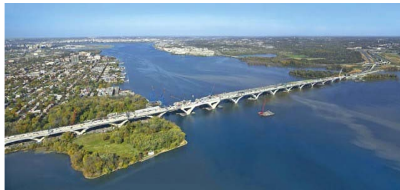
Figure 5.3.8: Concrete V-Piers (Woodrow Wilson Bridge)
