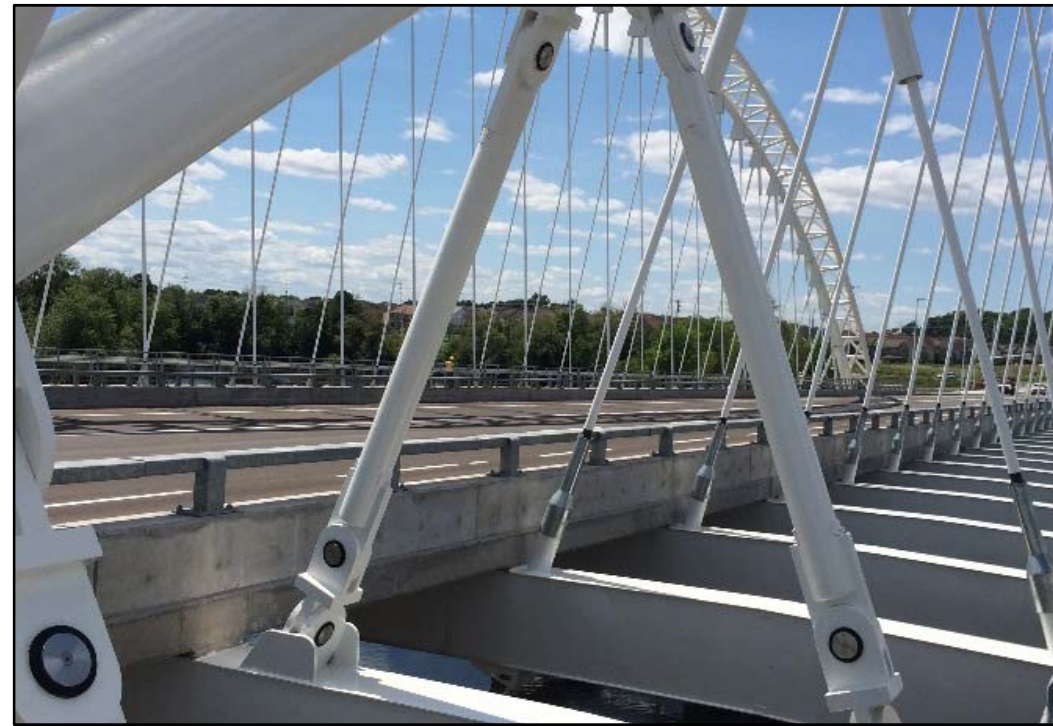
Figure 8.7.4.1: Low Wall Concrete Barrier with Steel Railing (Vimy Memorial Bridge)
