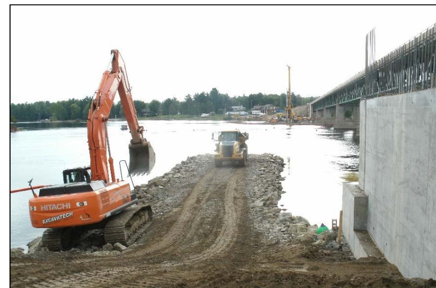
Figure 6.3.1: Temporary Earth Berm
