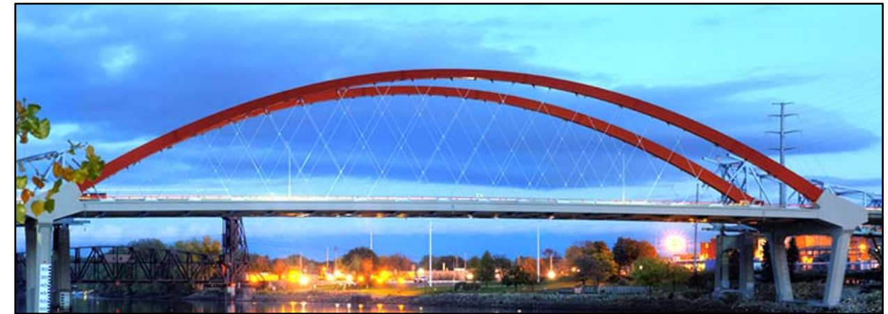
Figure 5.3.4: Network Tied Arch (Hastings Bridge)
