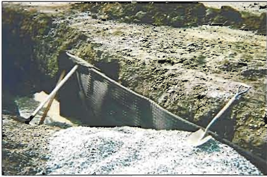
INSTALLATION OF TYPICAL PERIMETER LEACHATE COLLECTION TRENCH - DETAIL
