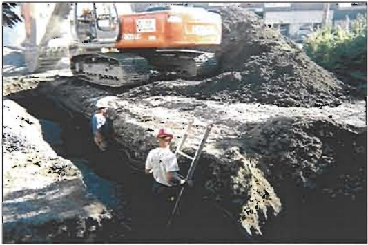
INSTALLATION OF TYPICAL PERIMETER LEACHATE COLLECTION TRENCH
