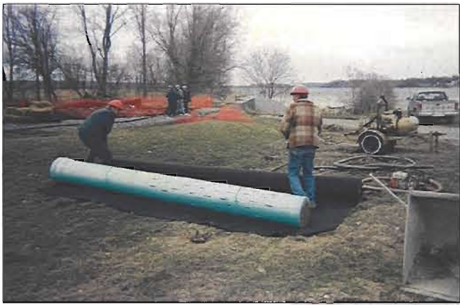
INSTALLATION OF TYPICAL PERIMETER LEACHATE COLLECTION PIPE
