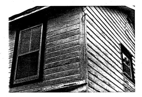
Wood siding must be kept weather tight. Regular cleaning and painting will be necessary to preserve this form of cladding.
