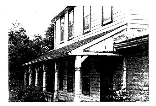
A proper roof inspection should be carried out annually. Sound flashing and operational downspouts and gutters are critical to the long term maintenance of this feature whether it is built of wood, metal or asphalt. around the chimney and dormers are often vulnerable and apt to fail. Remove affected metal and replace in kind. When sealants have failed due to expansion, age or improper application clean all surfaces and replace sealants as directed.
