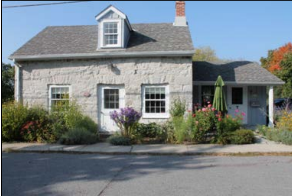
Photo 11: Example of a contemporary addition that is set back from the original building, located to the side, and compatible with the historic built form.
