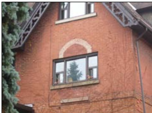
Photo 5: Changes to original window openings, as in the example above is not permitted.
