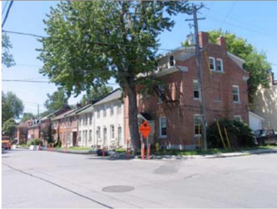
Streetscape view from William Street
