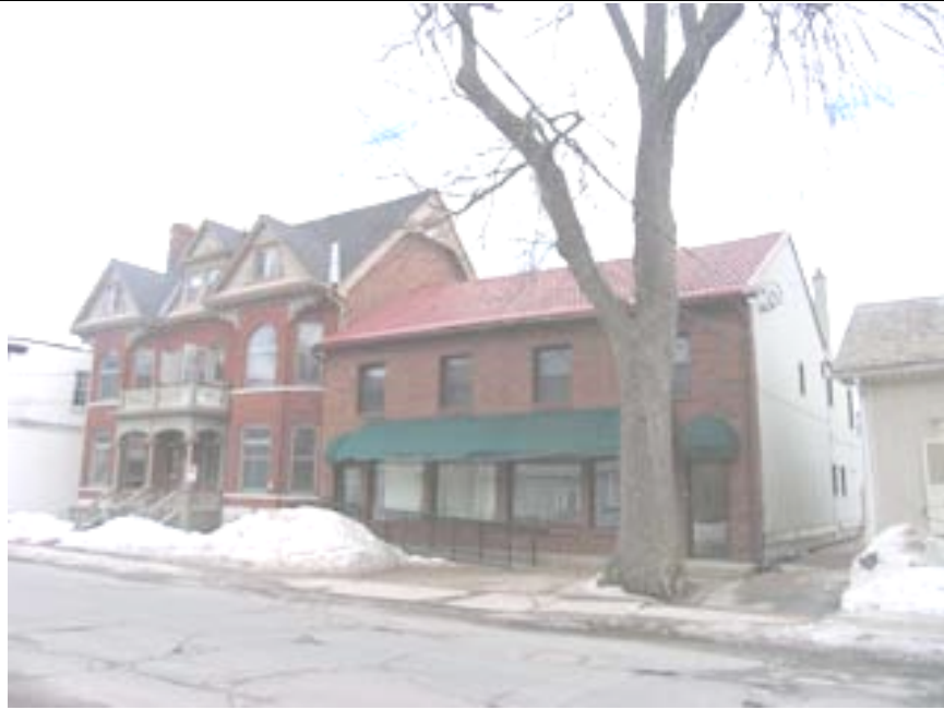
Streetscape view from southwest
