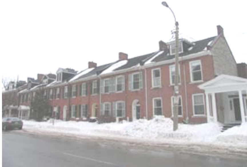
The full terrace from the northwest
