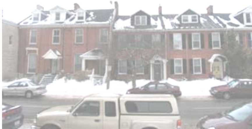
Partial streetscape view
