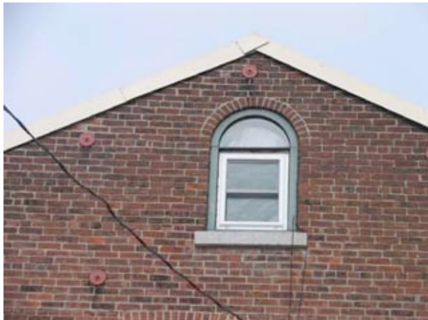
Arched window with rowlock voussoirs. Note wall ties and common bond brickwork
