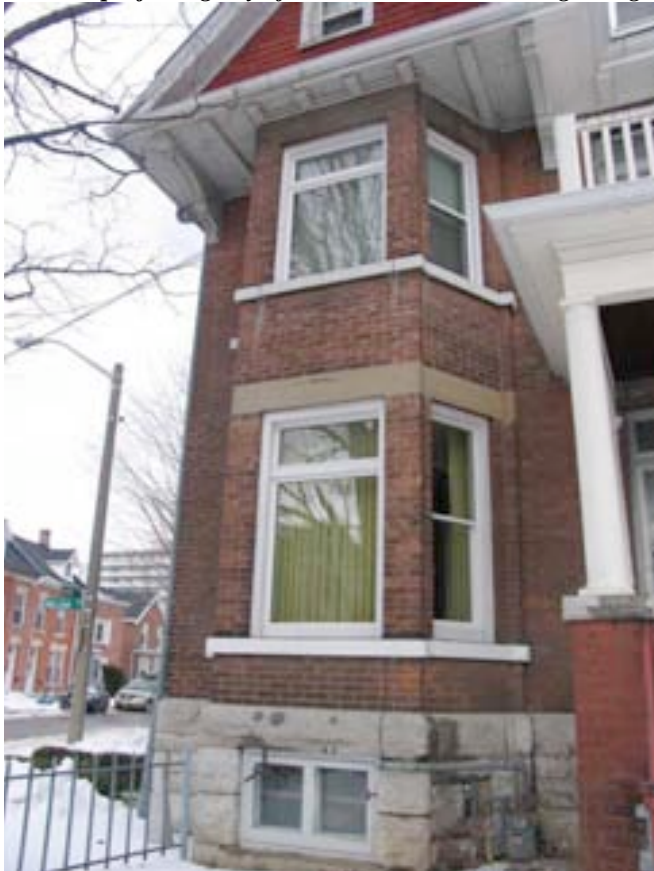
Detail of soffit at base of cross-gables Detail at projecting bay of 215 William. Note the right angled return at each section.
