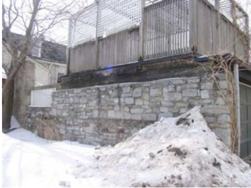
Section of original garden/boundary wall
