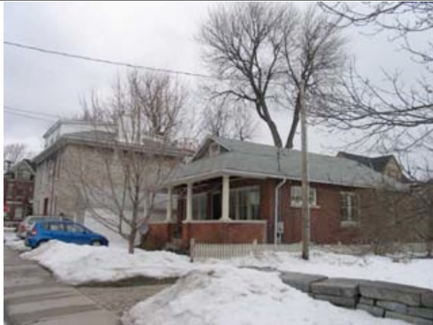
Streetscape view looking northwest
