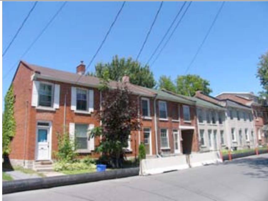
Streetscape view from southwest
