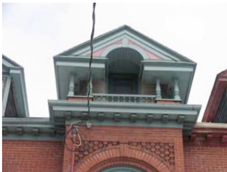
Detail of spandrel brickwork and unbraced cross gable
