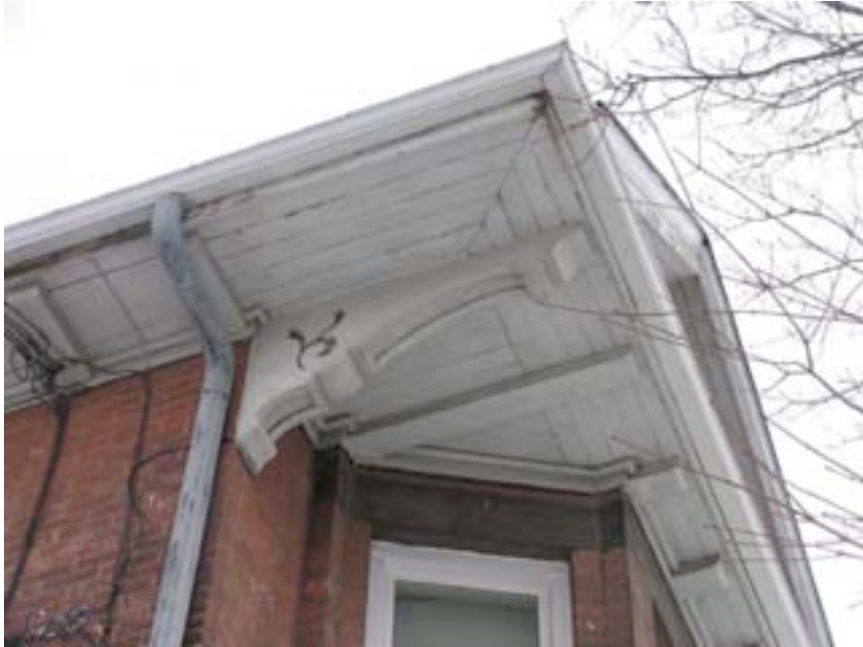
Detail of soffit at base of cross-gables Detail at projecting bay of 215 William. Note the right angled return at each section.
