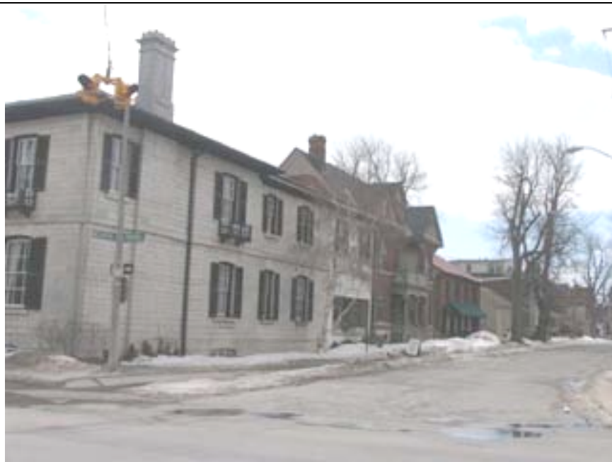
Streetscape view from northwest
