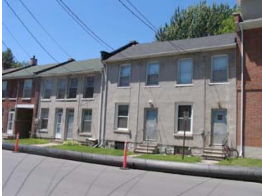
Streetscape view from northeast
