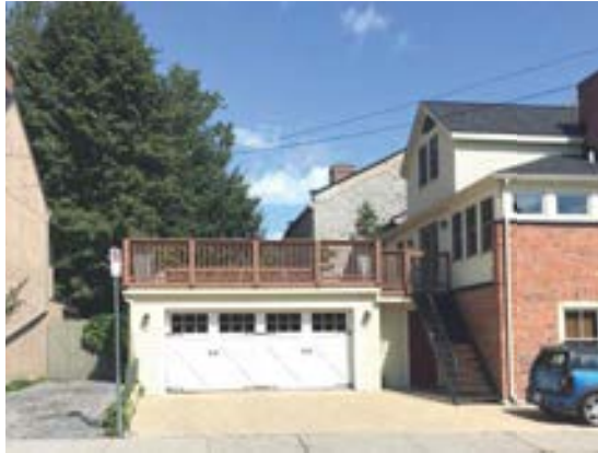
PHOTO OF EXISTING
