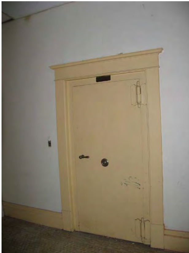
Detail: J & J Taylor Vault, 21 Queen St. (D26)
