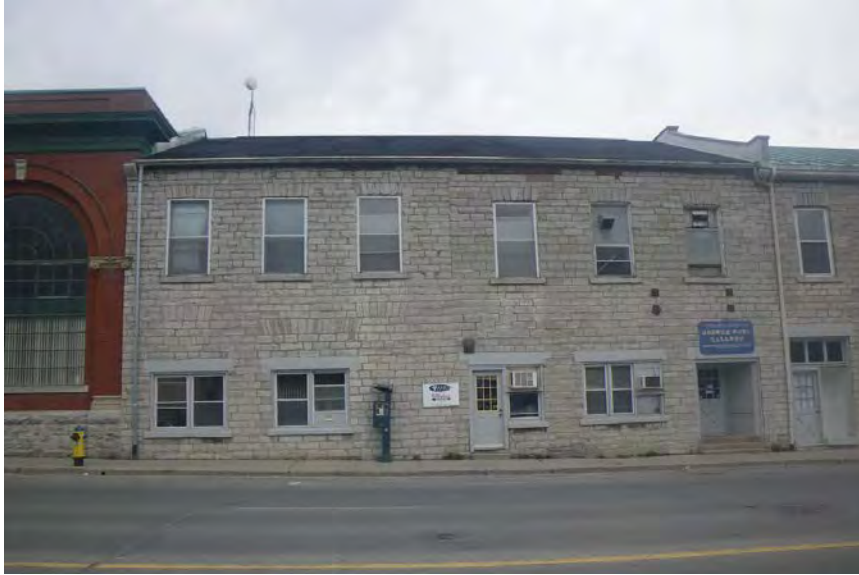
Partial view of façade – Western Section (GV1-06)
