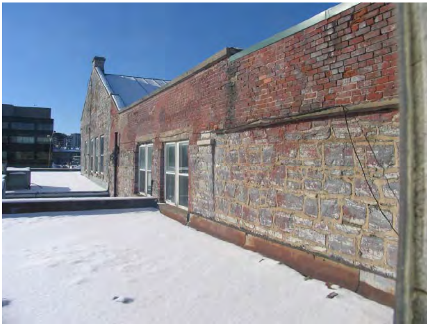
East Elevation – upper wall and later brick parapet (GV6-06)
