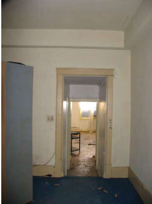
Detail: Typical door casing and base, 19 Queen St. (D31)
