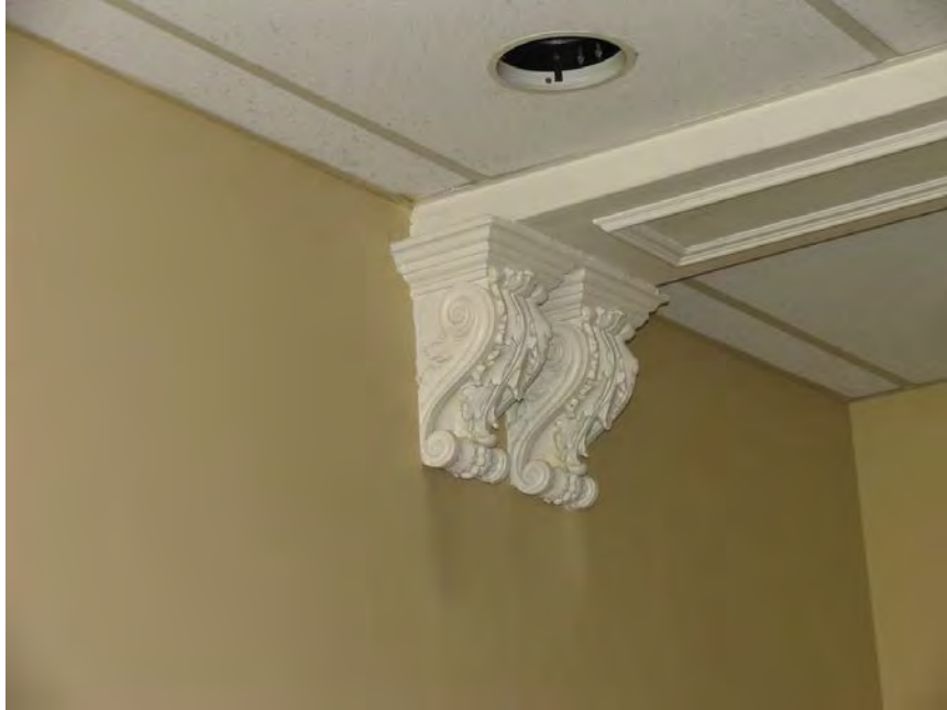
Detail: Panelled beam and ornate corbels in fibrous plaster, 19 Queen St. (D23)
