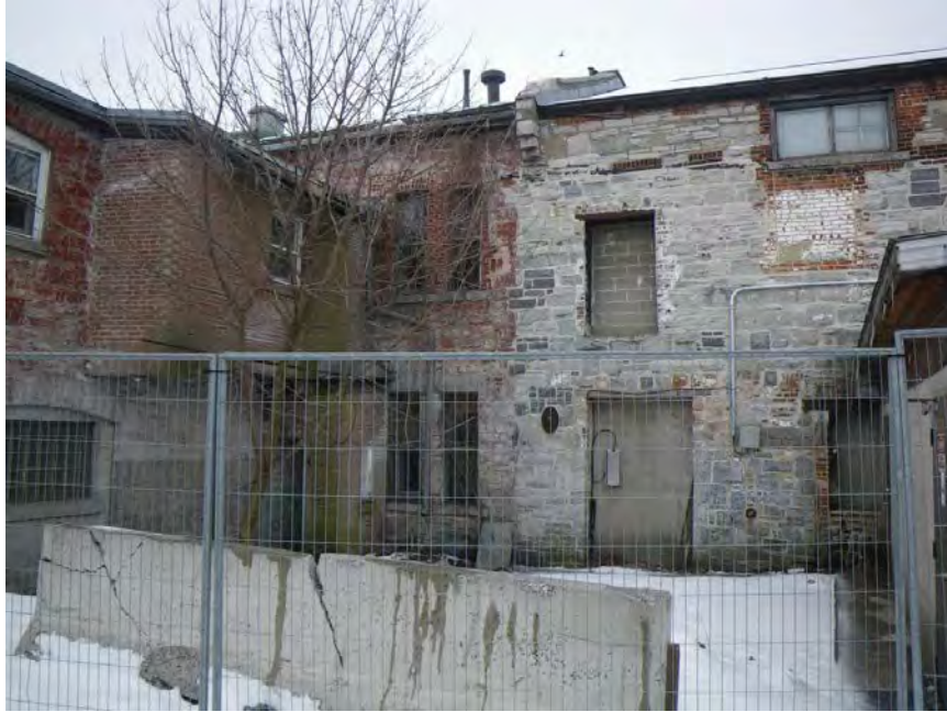
Partial view - North elevation including former carriage exit (D19)
