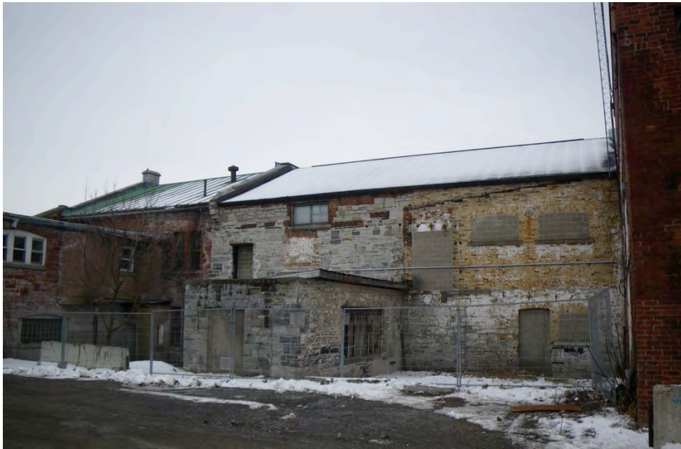
Fig.10: North elevation (except rear wall of rear addition) and 19 Queen St.
