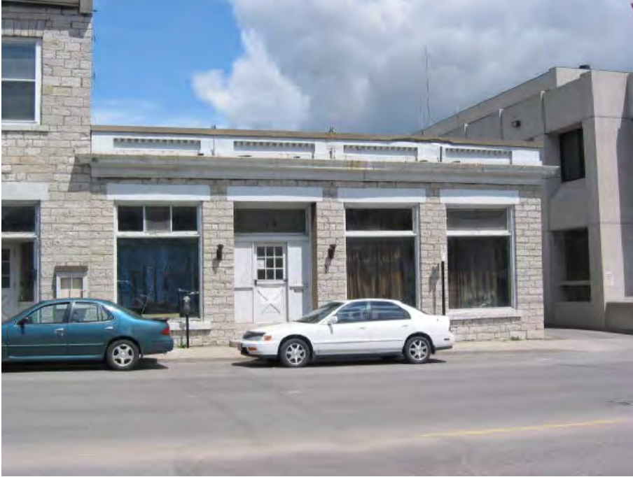
Fig. 8: 19 Queen St. Note lane at former Police Station (now demolished)
