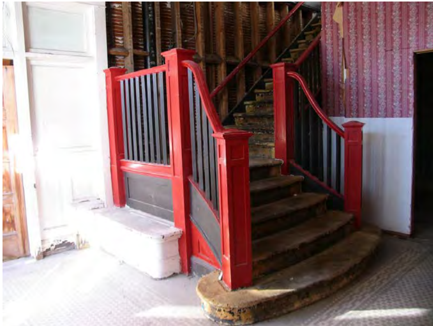
Detail: Staircase, 21 Queen St. (D32)
