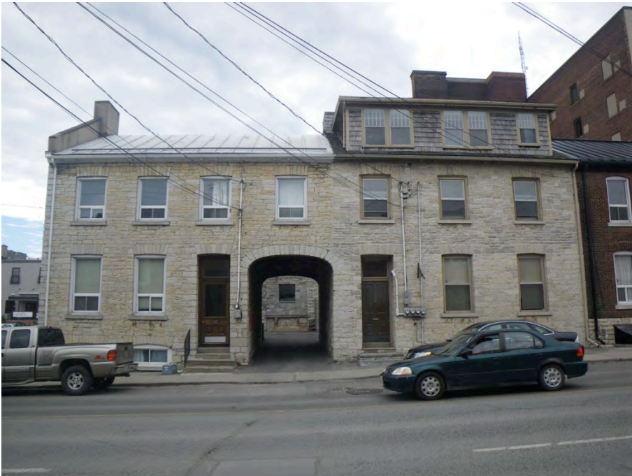
Fig.4: Detail of elliptically arched stone carriageway
