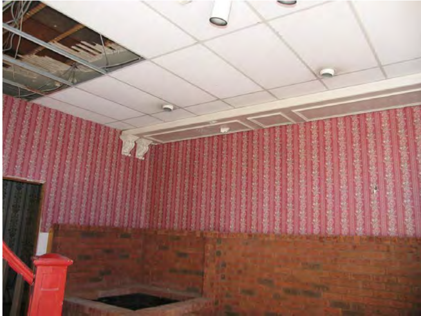
Detail: Fibrous plaster beam, 21 Queen St. (D29)
