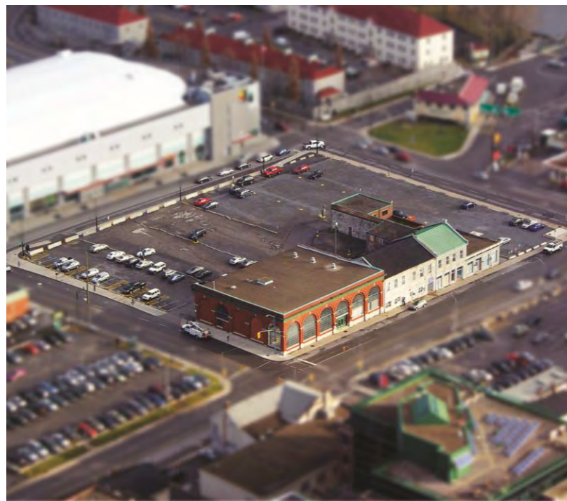
Photo 4: Existing structures on Block 4 including the Kingston Hydro substation and heritage buildings at 19, 21 and 23 Queen Street
