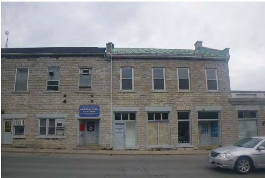
Partial view of façade – Central Section (GV2-06)
