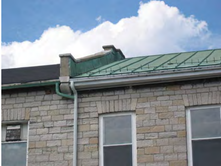
Detail: Stone parapet and corbel (D2)
