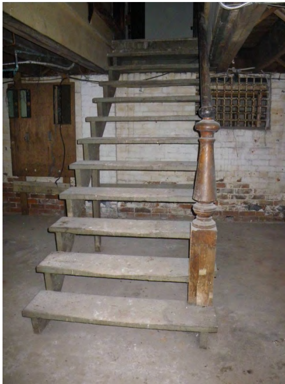
Detail: Basement stair rail and newel (D35)
