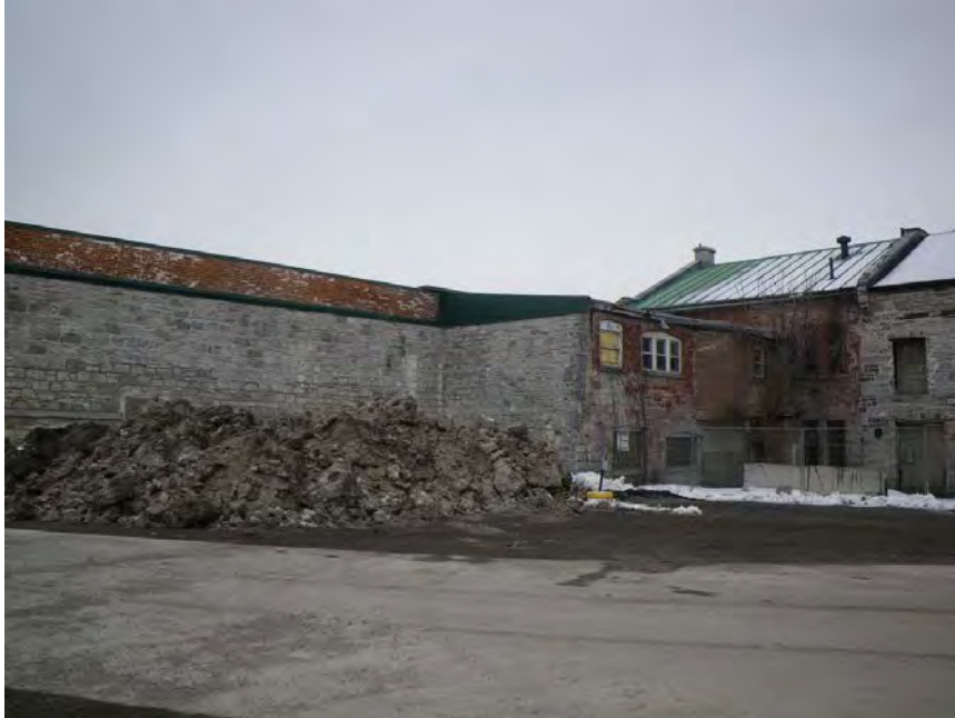
View of early rear addition and surviving gas-holder wall (GV1-07)
