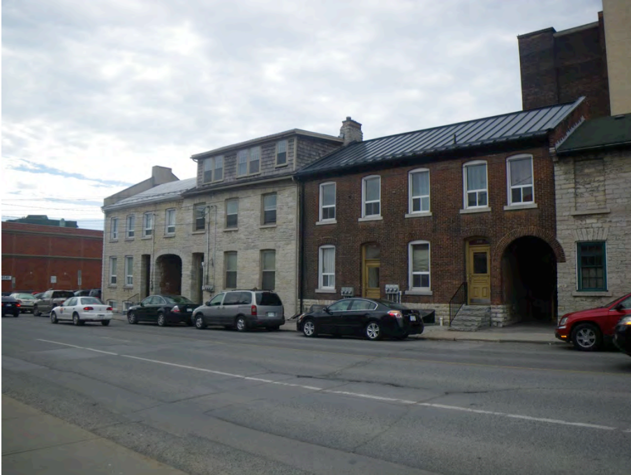
Fig.3: Arched carriageways at Queen St. east of Bagot St.
