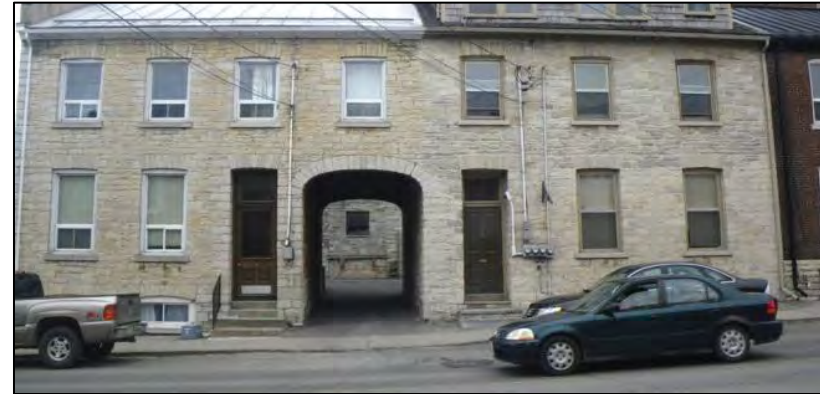
Photo 13: Existing Carriage Way, Kingston
