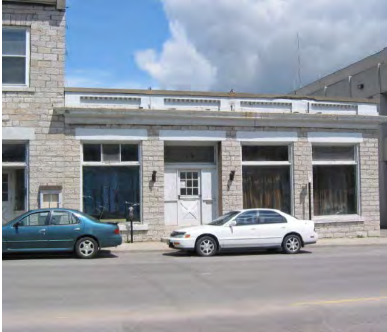
Partial view of façade – Eastern Section(GV3-06)
