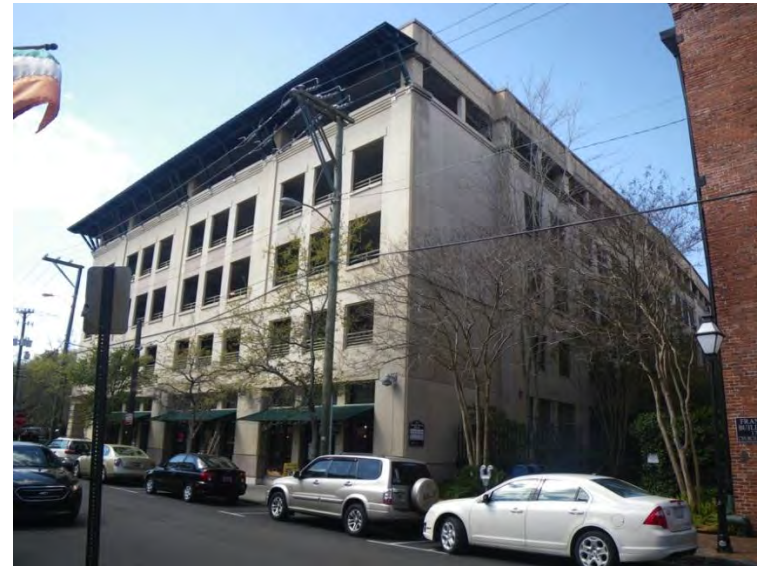
Photo 20: Parking garage with architectural screening, Charleston
