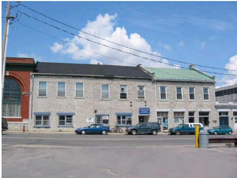
Fig.1: Existing façade 21-23 Queen Street
