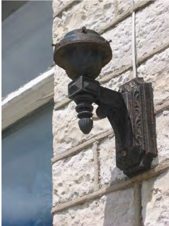
Detail: Surviving original gaslight sconce (D12)
