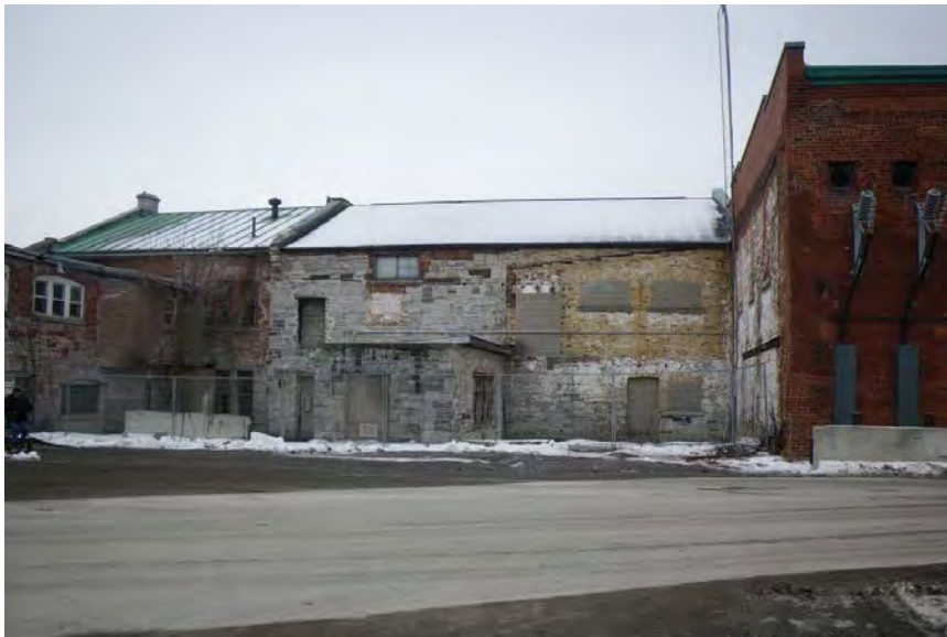
General view – North Elevation (GV2-07)
