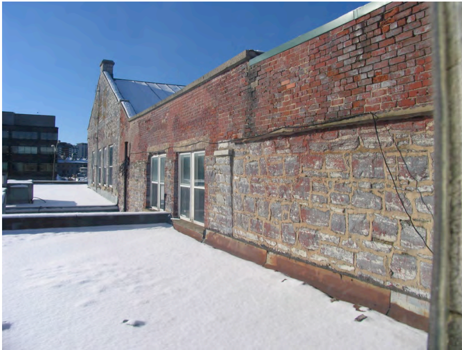
Fig.9: Upper wall of rear addition- brick parapet above original stone
