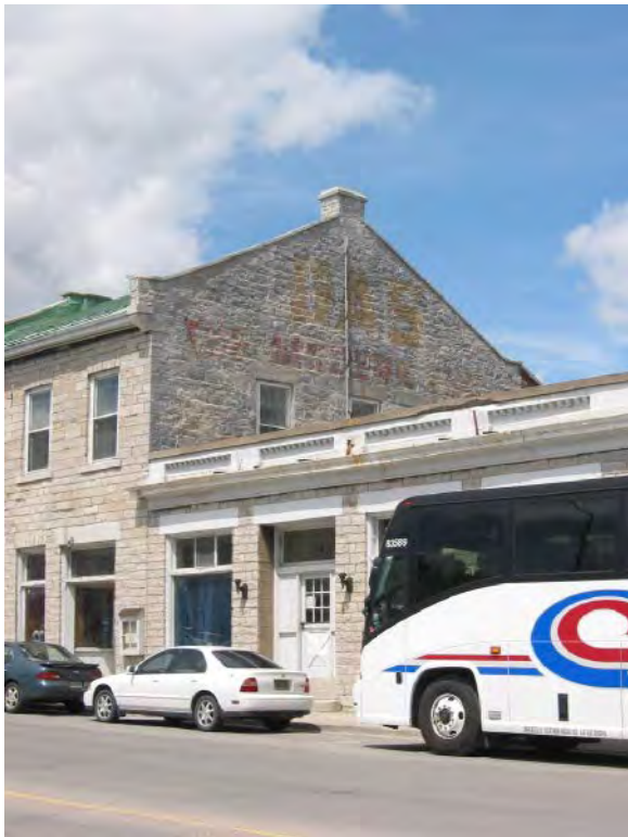
East gable with 'Modern Gas' signage (GV4-06)
