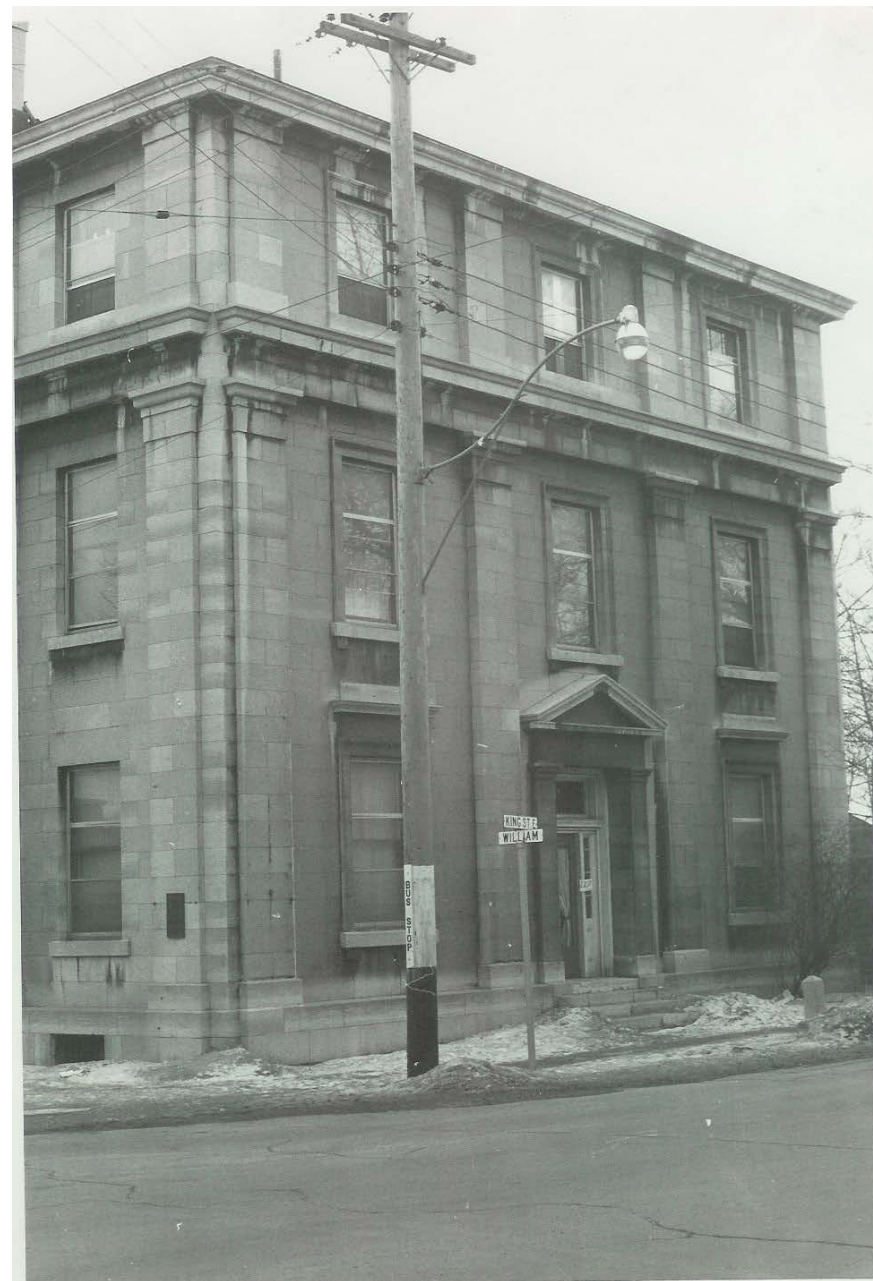
Historic Photograph - Front Elevation from King St. E.
