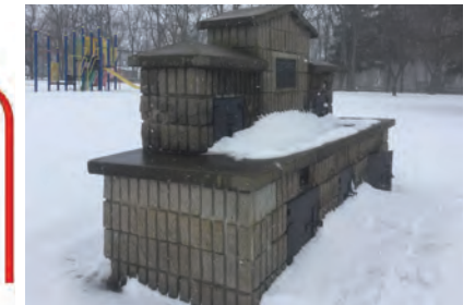
Existing BBQ to be removed
