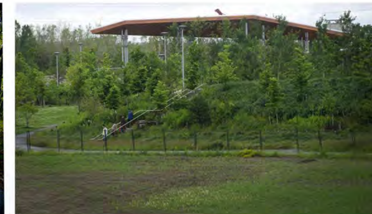
Naturalized Berm Planting
