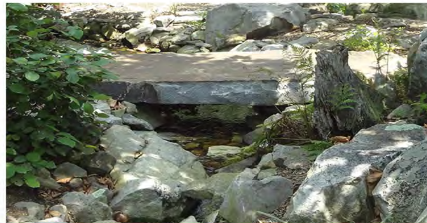
Stone Slab Bridge
