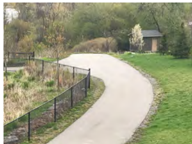
Existing Asphalt Path Leading to Existing Woodland
