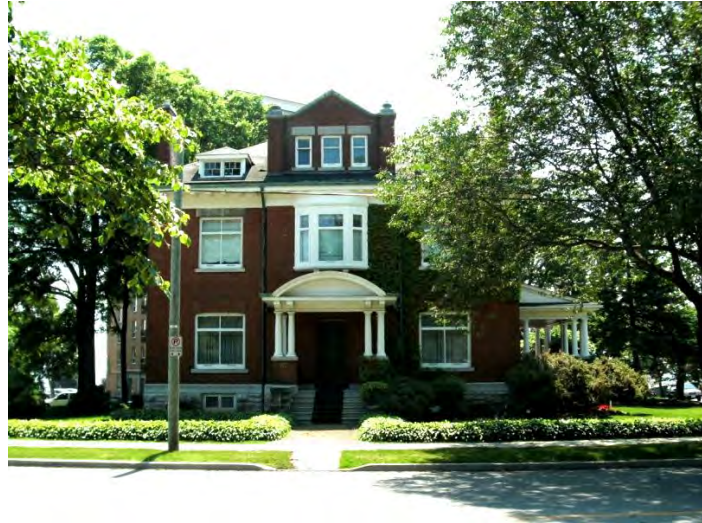
Façade, viewed from King Street East
