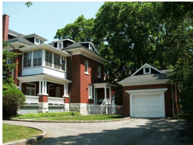
Southeast elevation from Simcoe Street
