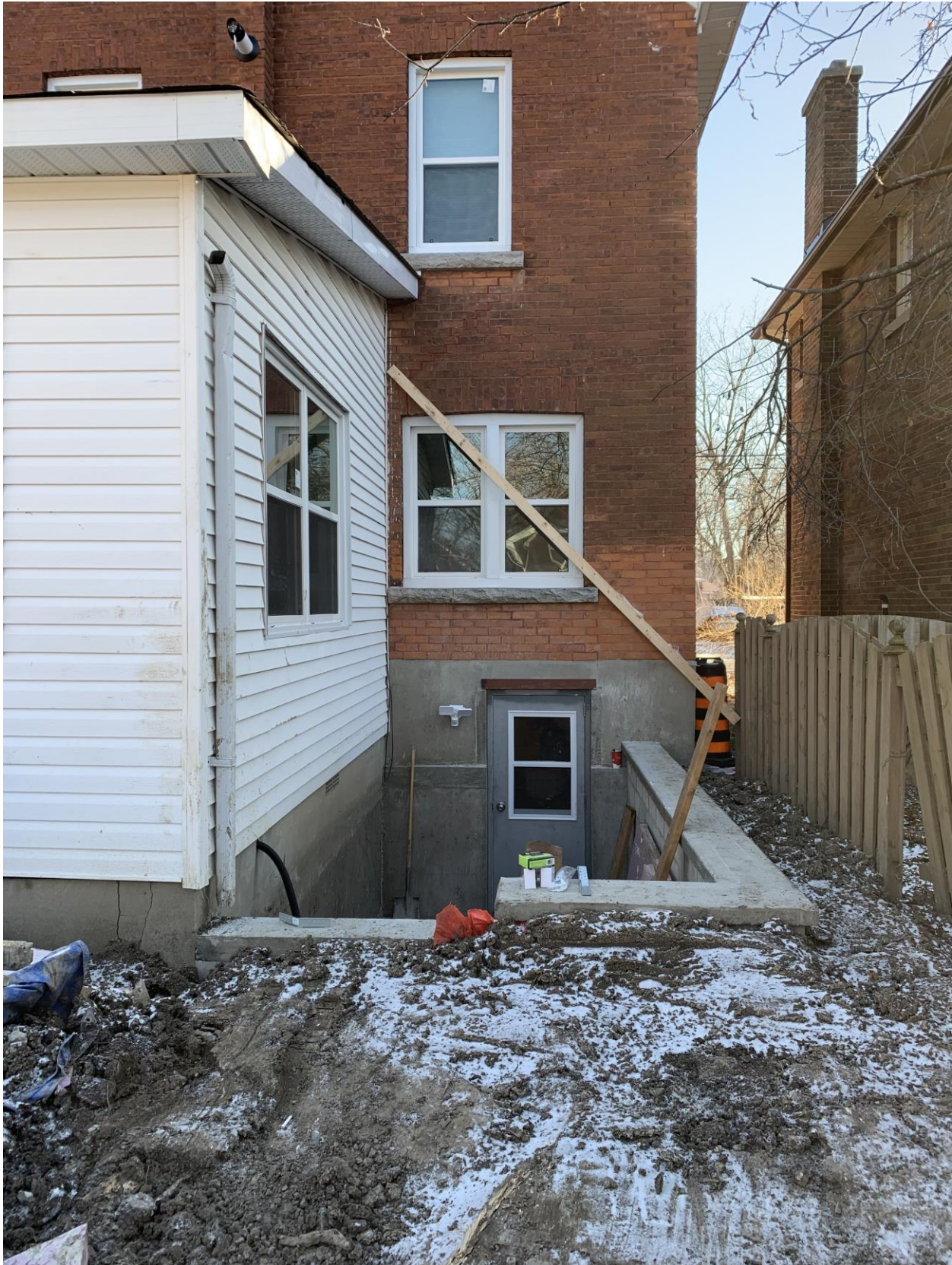
Rear Entrance - Context photograph submitted by applicant
