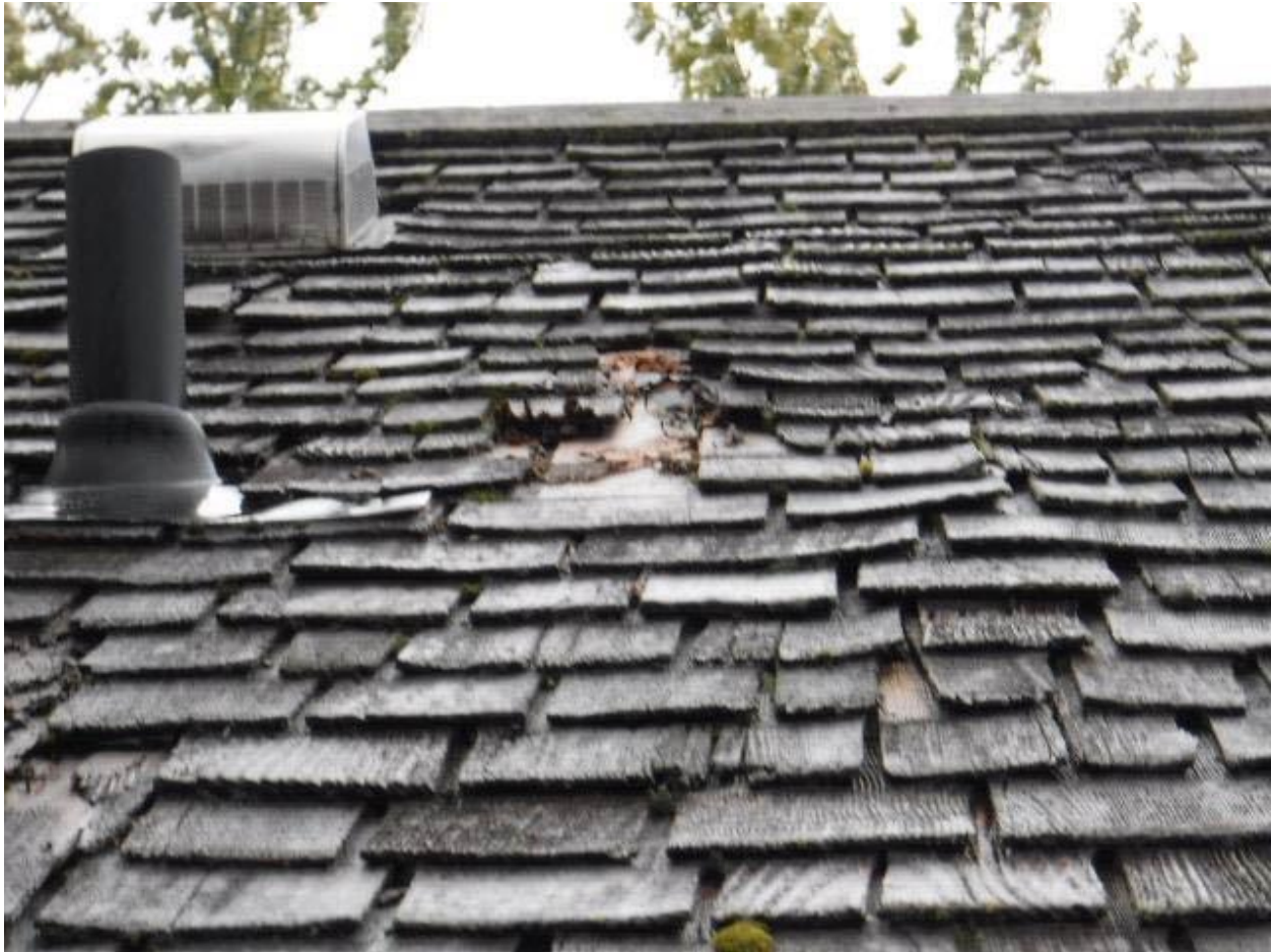
Photograph of Roof Submitted by Applicant
