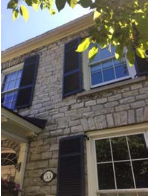
Figure 6: North wall of subject property
