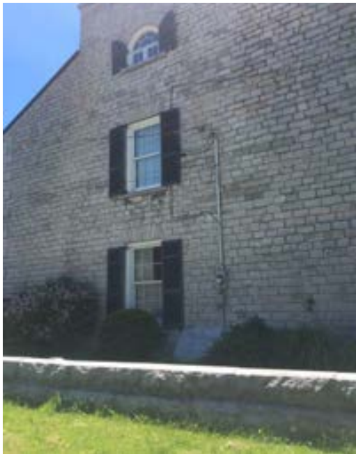
Figure 3: East wall of subject property
