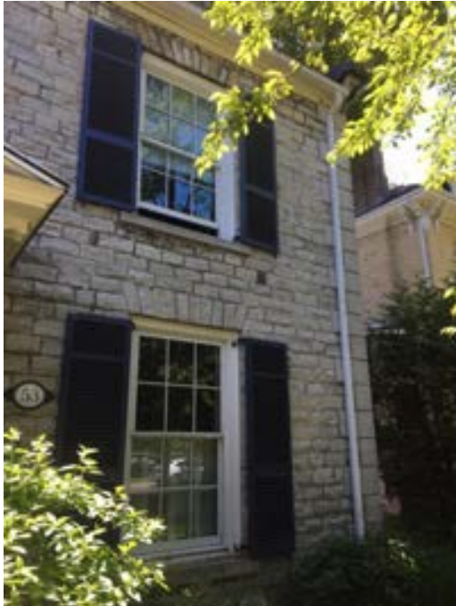
Figure 1: North wall of subject property
