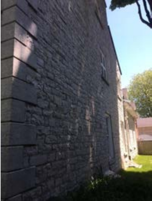
Figure 5: West wall of subject property
