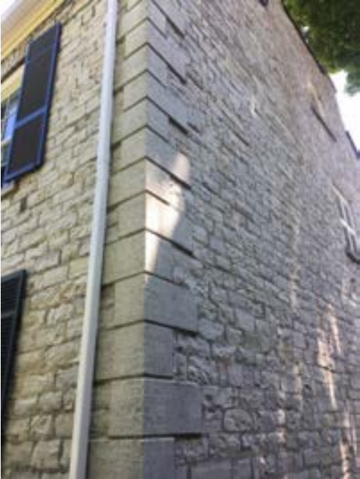
Figure 7: Northwest wall of subject property
