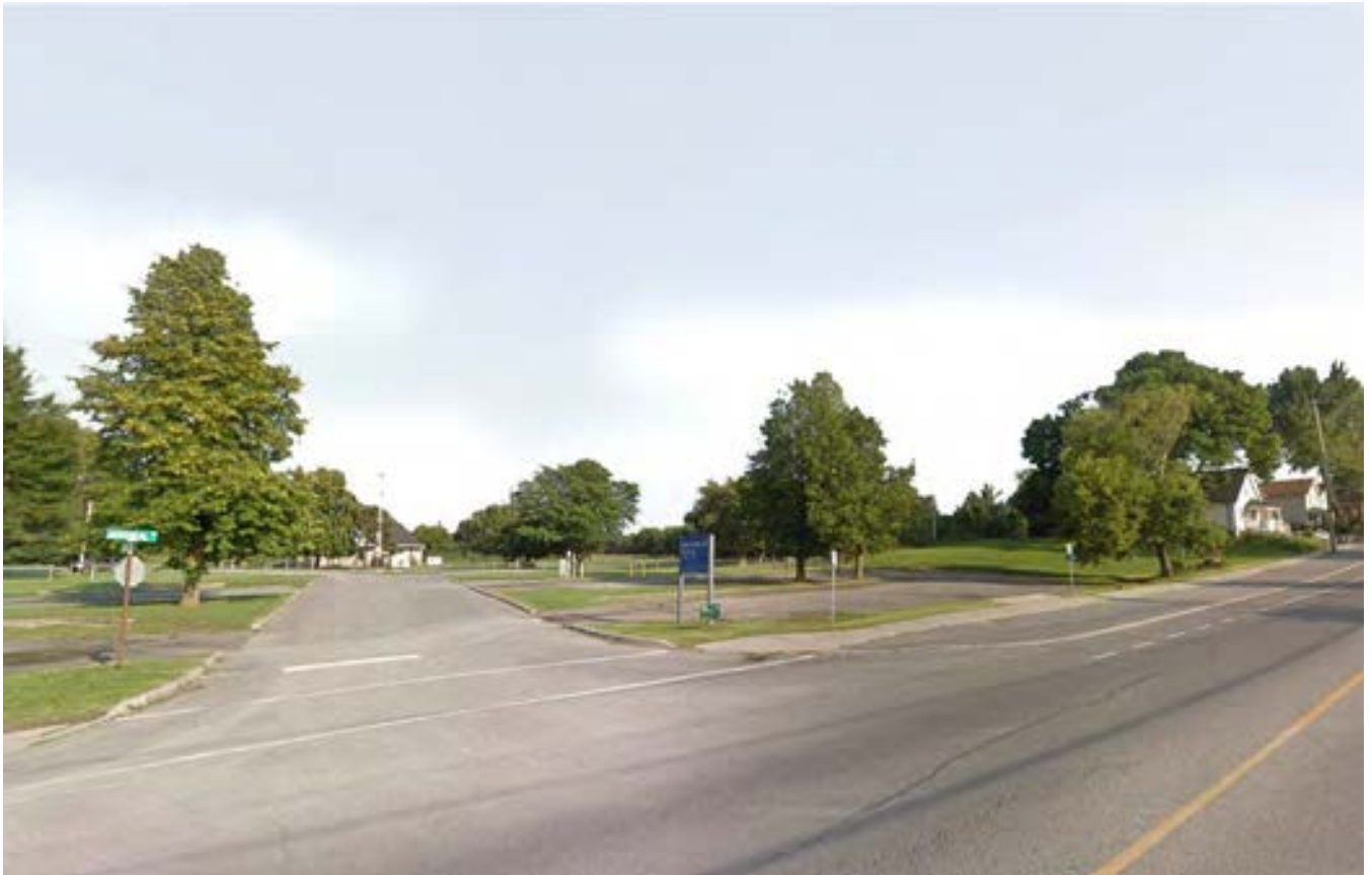
BEFORE: Current Gateway Entrance
