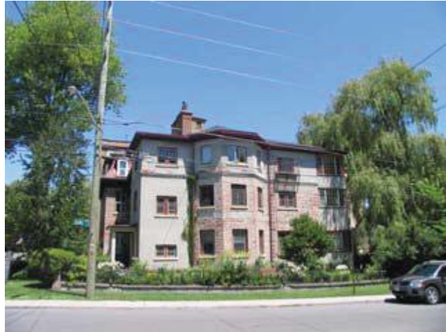
Carruthers Villa with additions; view from southwest
