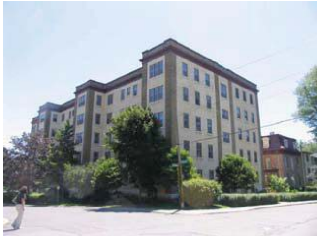
The Annandale Apartments; view from northwest
