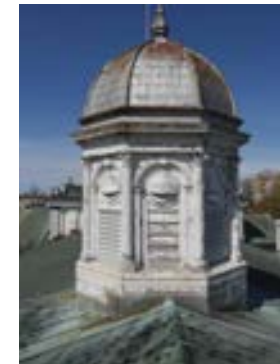
IMG 03: EXISTING EAST CUPOLA (2017)
