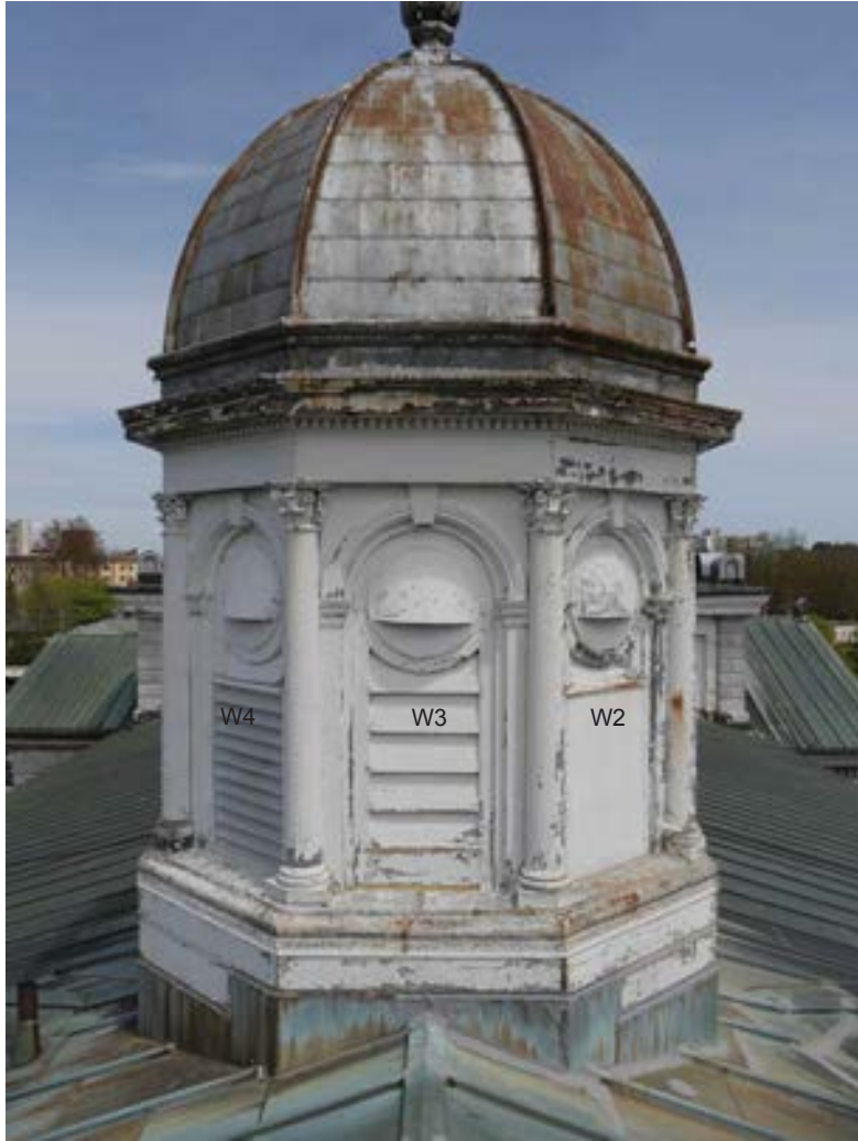
1 PHOTO - W. CUPOLA ELEVATION: VIEW SHOWING EXISTING CONDITIONS A005 N.T.S.
