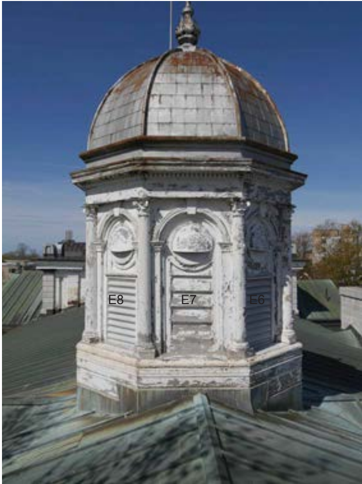
1 PHOTO-E. CUPOLA ELEVATION: VIEW SHOWING EXISTING CONDITIONS A003 N.T.S.
