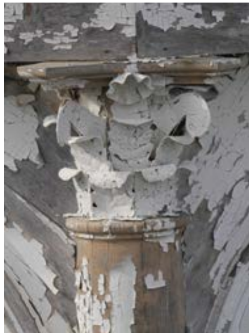
Fig. 31 East cupola . Typical example of metal details at the Corinthian capitals (THA 2017).
