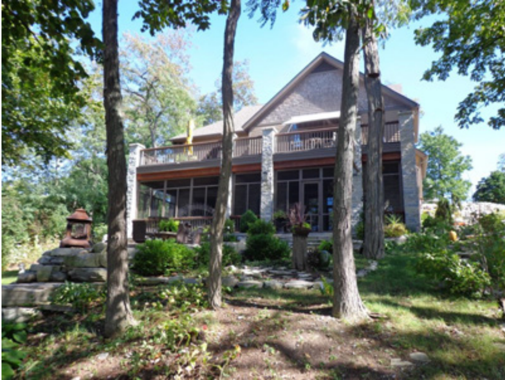
Figure 3: View of the scope of work area from the sloping hill.
