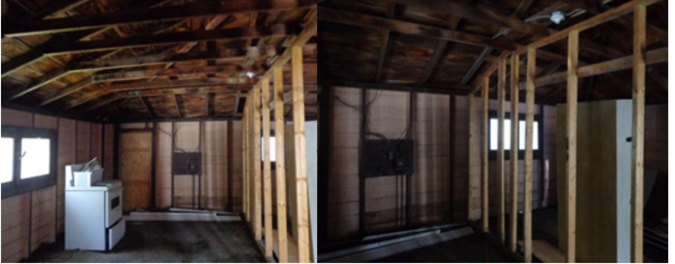
Figures 8 and 9: Interior of garage.
