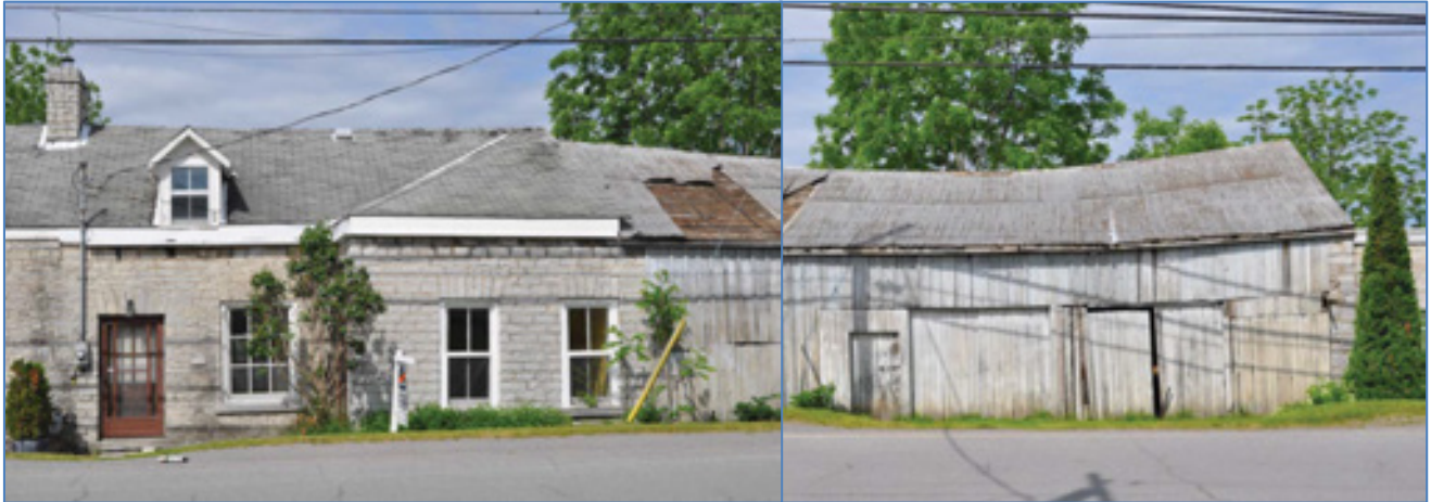
Finley's additions of the 1860s digitally stitched together: the stone L-shaped section on the left and the frame (with stone rear and end walls) drive shed on the right (photo 2011, J. McKendry)
