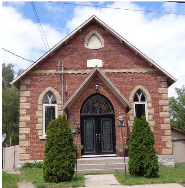
704 Hillview Road – former Collins Bay W. Methodist Church
