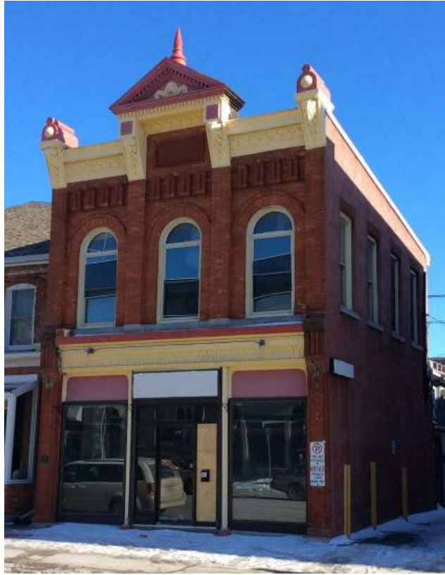
181 Sydenham Street – C. Gildersleeve Building
