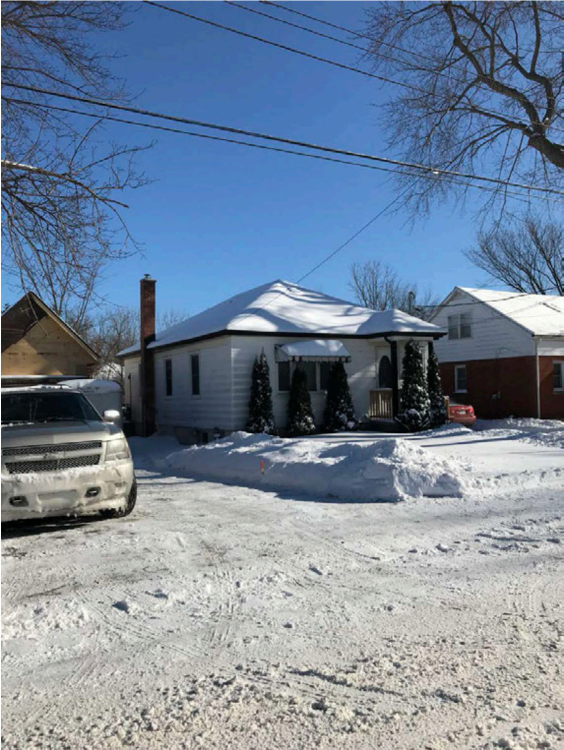
Figure 2: 339 College Street front elevation.
