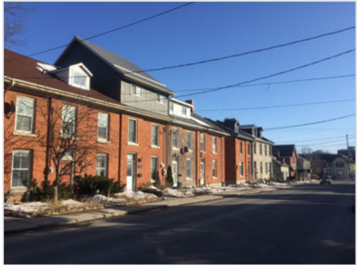
East side of Rideau Street looking south past subject property
