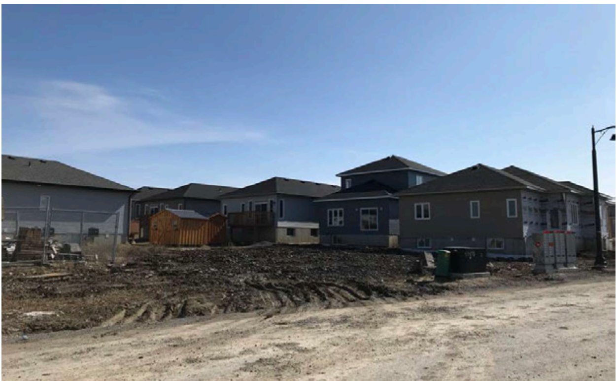
Figure 2: 1525 Clover Street existing Carfa Crescent street frontage.
