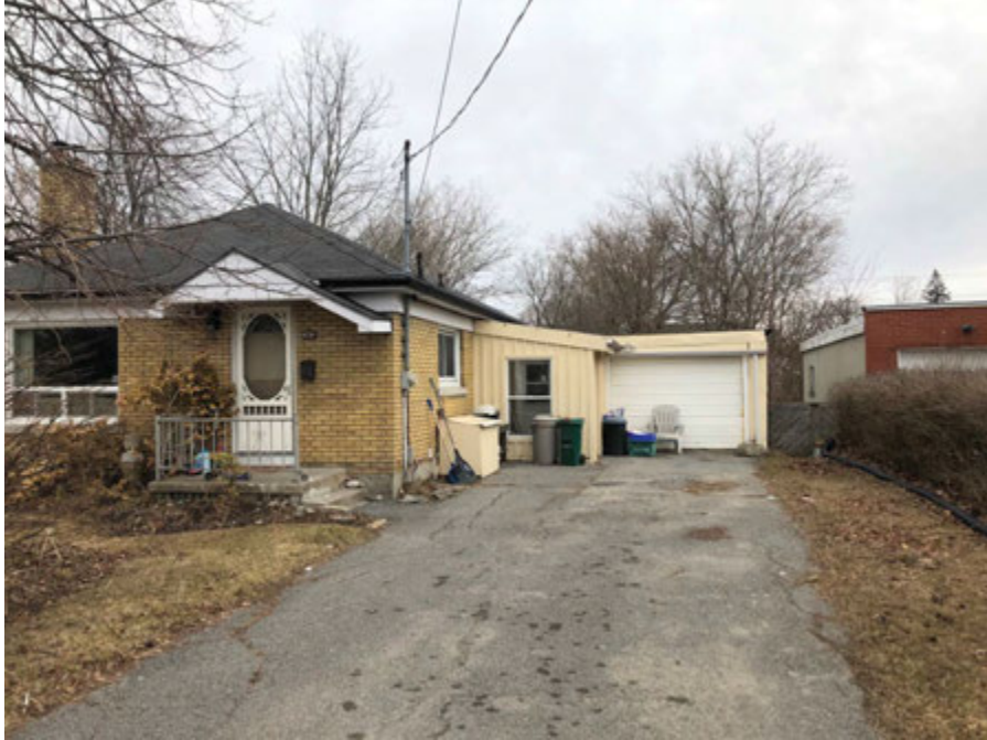
Figure 1 - 363 College Street Facade
