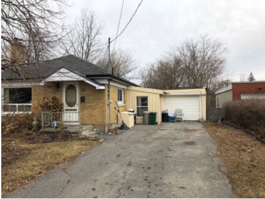
Figure 1 - 363 College Street Facade
