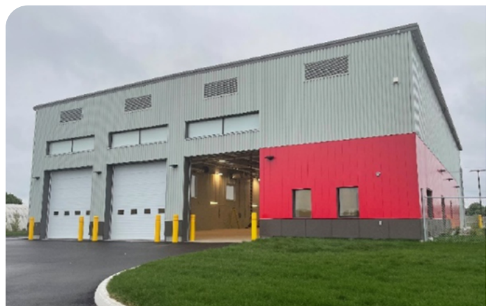
Figure 2: Kingston Fire & Rescue Maintenance Garage
