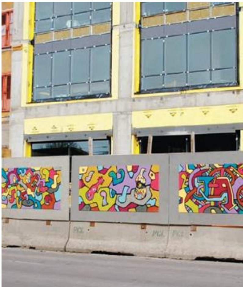
Enhanced Hoard, City of Calgary
