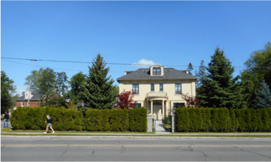
Fig 3: Front view of property
