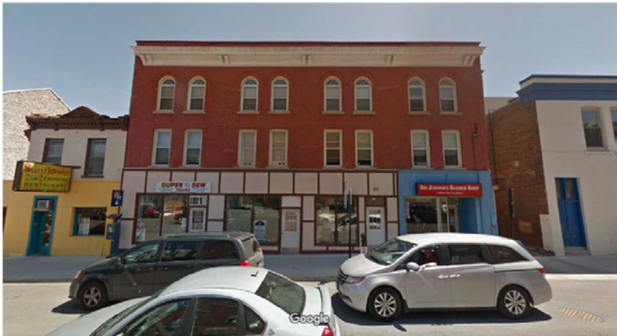
Figure 1: 35 - 39 Montreal Street, as seen from Montreal Street
