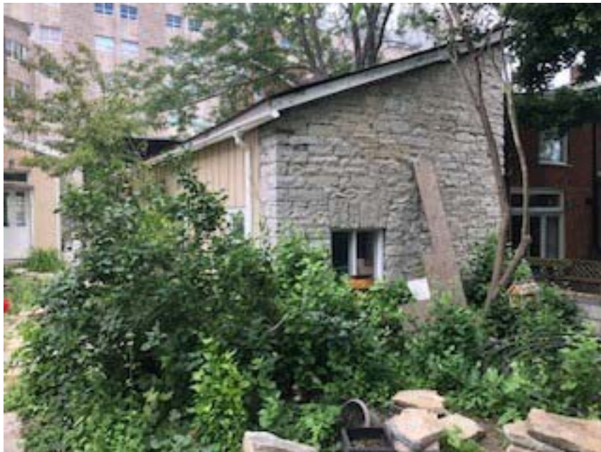
Figure 4 - Rear of Garage
