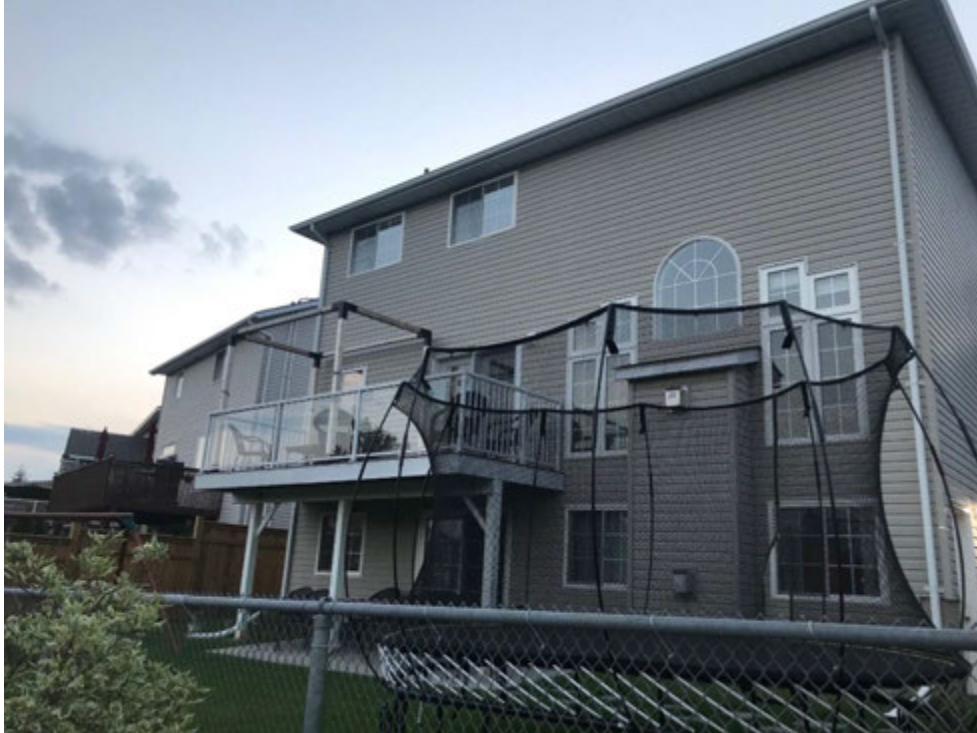
Figure 3 - View of Rear of Dwelling
