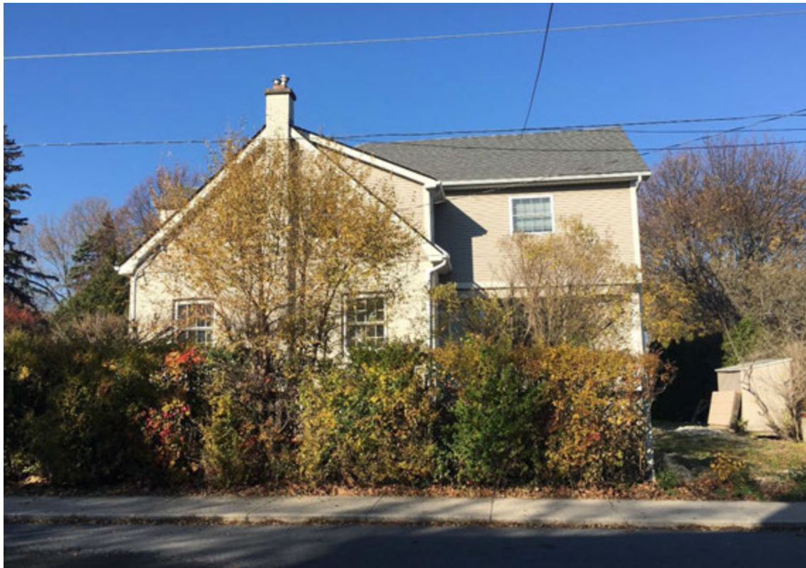
Figure 2: Existing two-storey dwelling Hill Street frontage.
