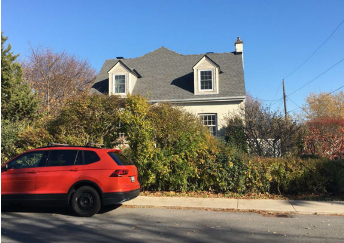
Figure 1: Existing two-storey dwelling College Street frontage.
