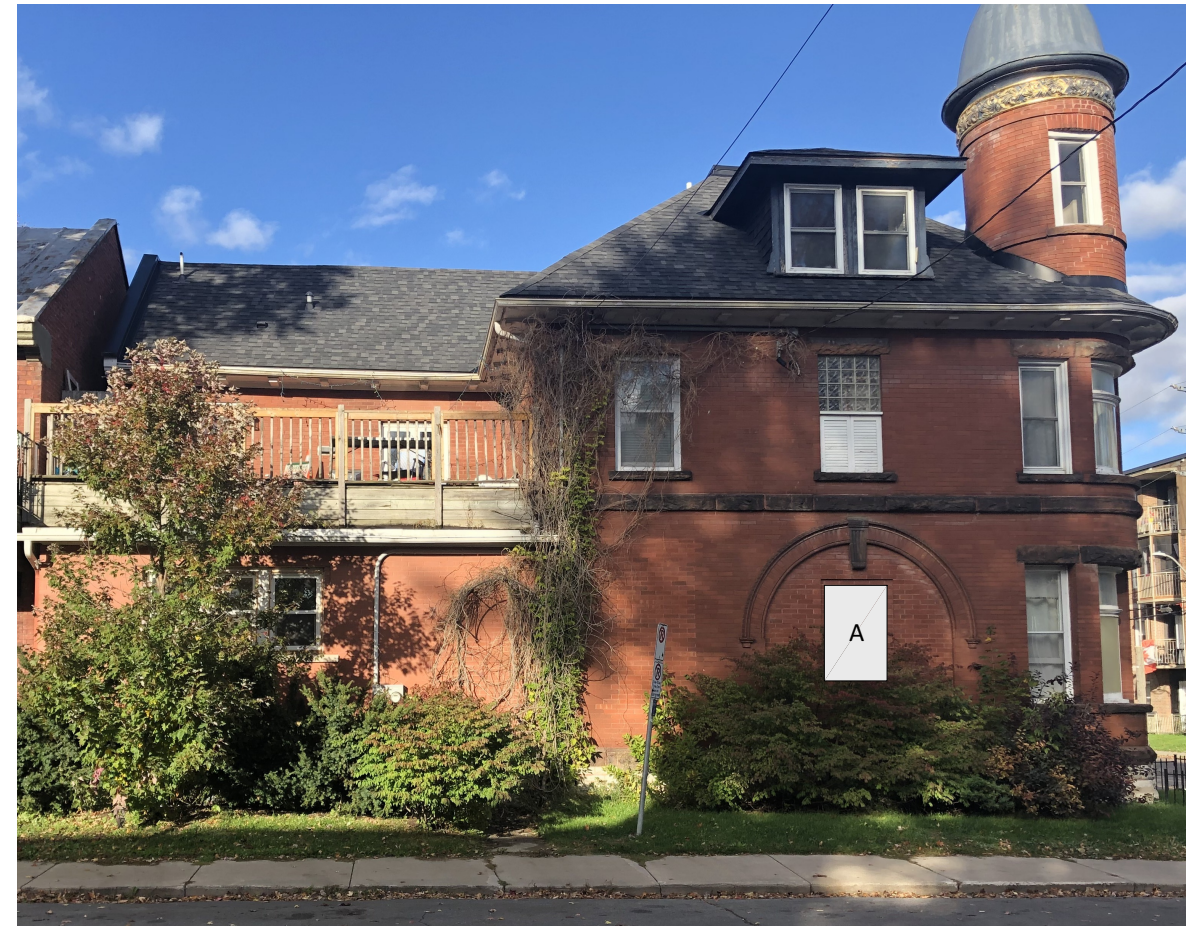
PHOTO of SOUTH WALL
