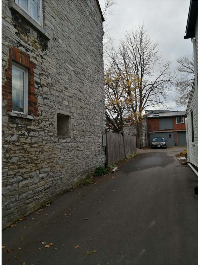
View from King Street.
