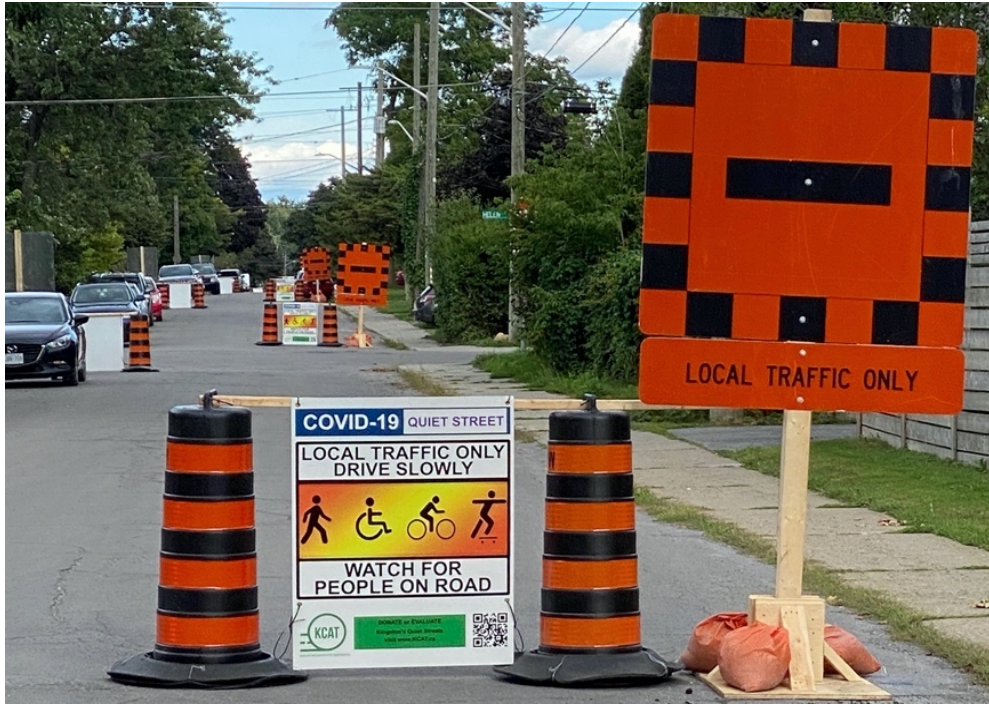
Figure 9: Newly installed traffic barriers along Mack Street of Quiet Streets route
