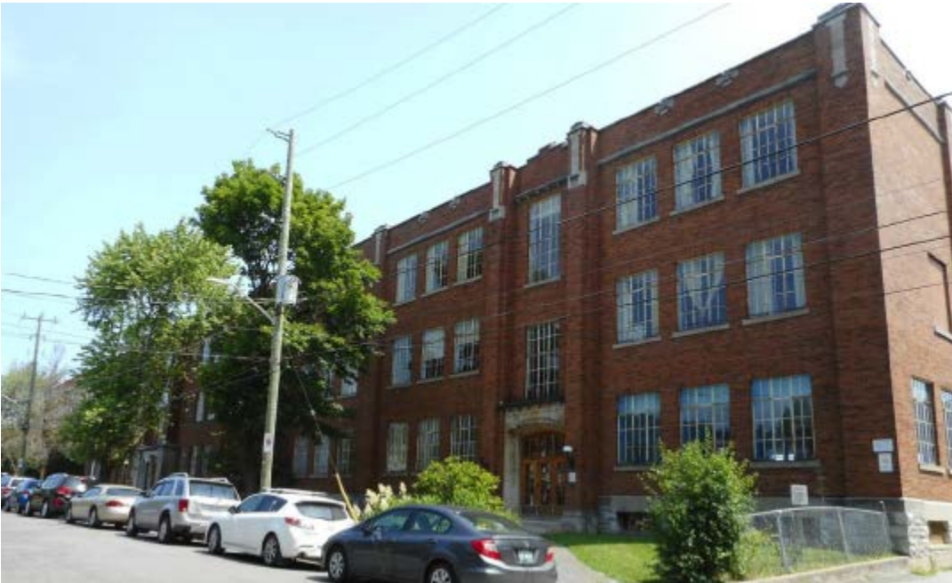
KCVI on the other side of the street
