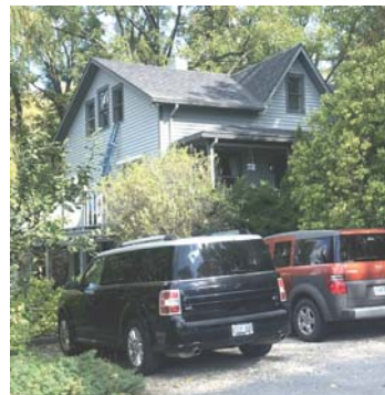
EXISTING VIEW FROM SOUTH WEST6
