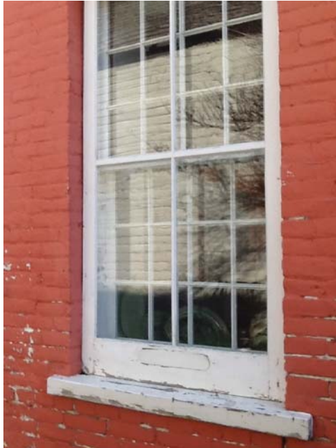
Sash Window with Storm on North Elevation
