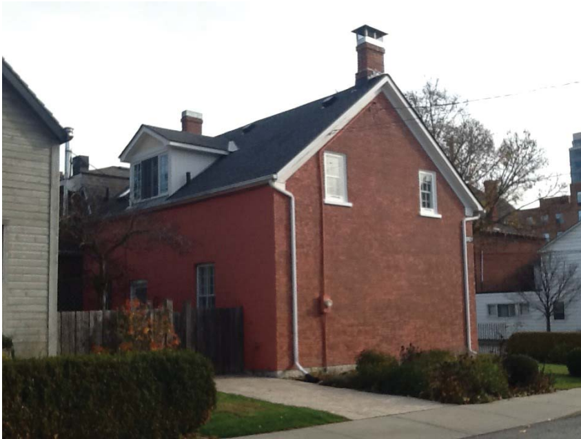
North and West Elevations (paint removed on West elevation)
