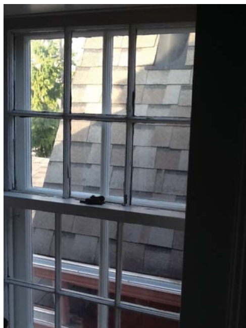
Interior of Sash Window on East Elevation
