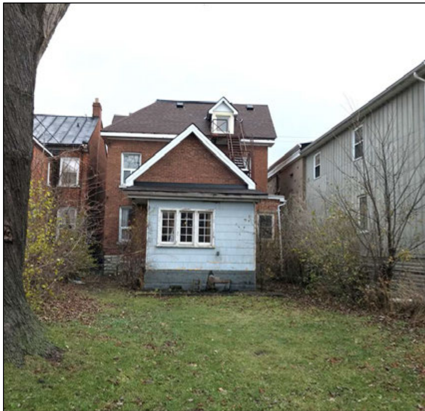
Figure 2: 370 Brock Street existing rear yard and one-storey rear addition.
