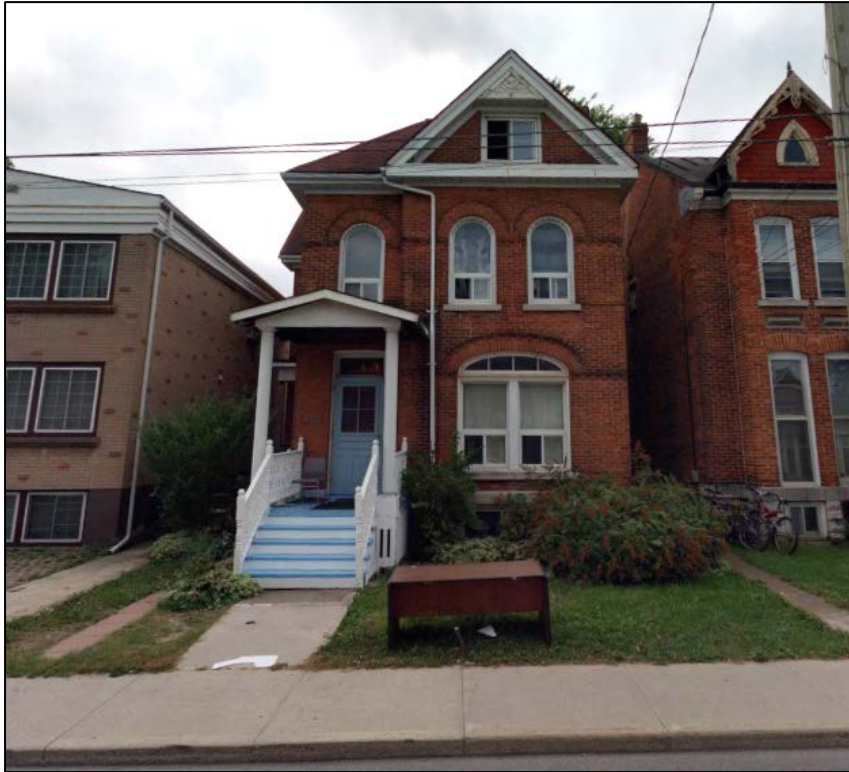
Figure 1: 370 Brock Street existing façade facing Brock Street.
