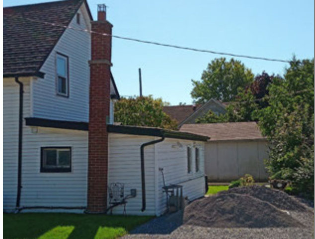
View of Garage from Wellington Street:
