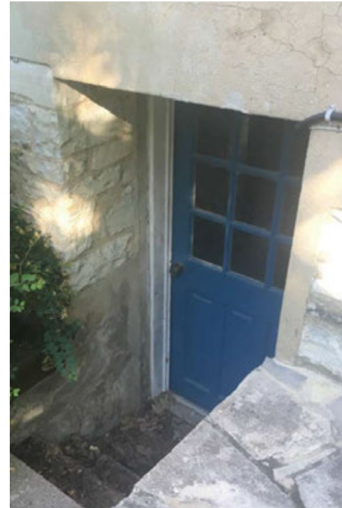
Garbage Room – to be retained and painted grey or black
