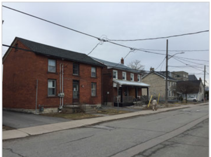
North side of Ordnance Street east of subject property.
