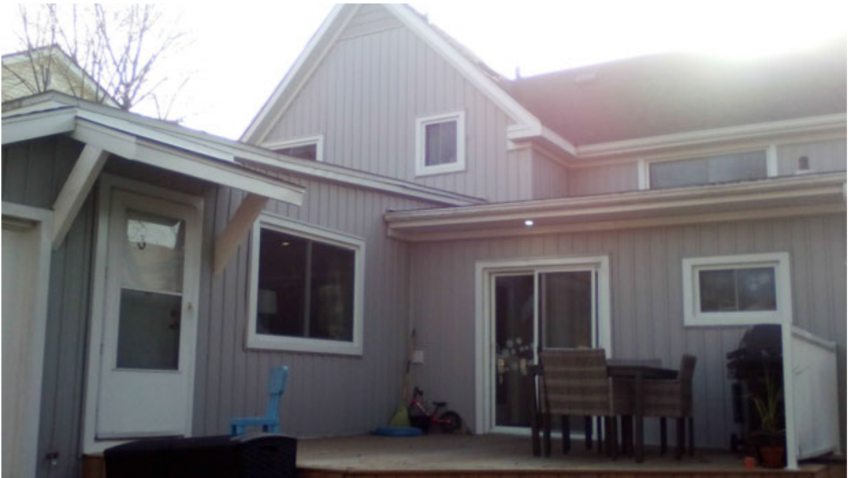
Rear of existing house at 585 Union Street, including the existing one-storey addition.
